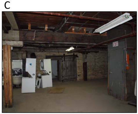
Looking towards Dundas Street – Existing Fire Door
