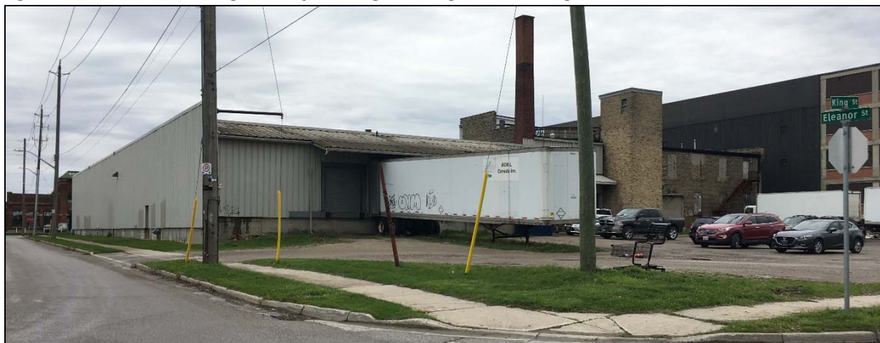
Figure 3 – Rear of the Existing 2-Storey Building (Looking North on King Street)
