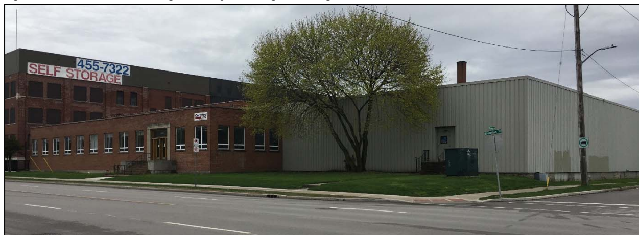
Figure 2 – Front of the Existing 2-Storey Building (Looking East on Dundas Street)
