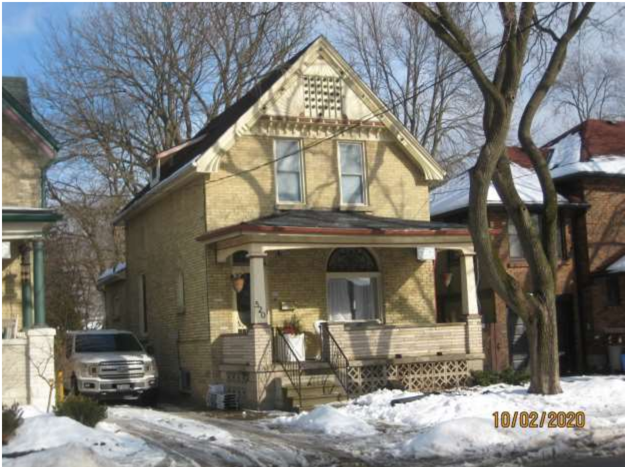
Image 9: Photograph of the dwelling located at 520 English Street within the Old East Heritage Conservation District, showing a set of second storey windows, similar to the proposed alterations at 512 English Street. Note, the decorative millwork in the gable of this dwelling extends to the tops of the windows, so voussoirs are not observed on this house.
