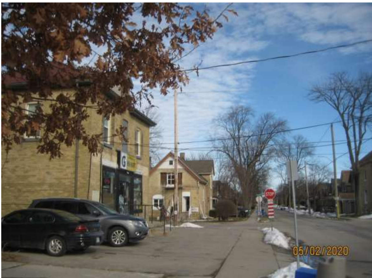
Image 2: Photograph showing the dwelling at 512 English Street, located at the corner of Lorne Avenue and English Street within the Old East Heritage Conservation District. Note, the proposed alterations to the dwelling are underway.
