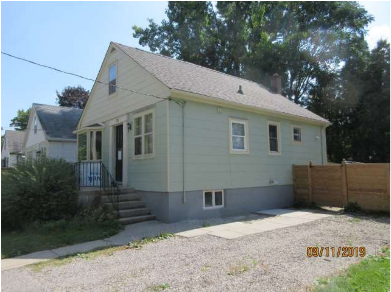
Image 3: View of the north (main) and west elevations of the dwelling located at 70 Rogers Avenue on September 11, 2019 (showing the completed alterations to the west elevation and the altered front window).
