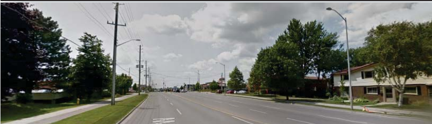
Looking west on Oxford St. W., west of Fiddler's Green Rd.
