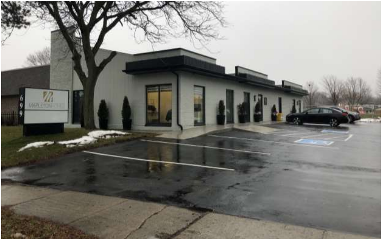
Figure 1: Existing building at 699 Village Green Avenue
