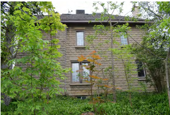
Plate 29: West façade of residence, looking east
