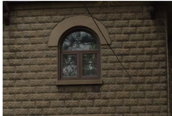
Plate 24: Second storey window on projecting gable bay, looking south
