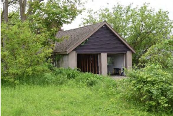
Plate 33: Garage, looking south
