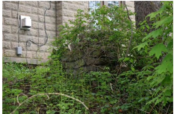
Plate 17: Rusticated concrete blocks, looking east
