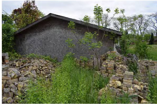
Plate 9: Buff brick piles, looking north
