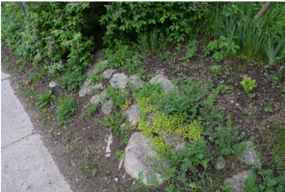
Plate 16: Concrete partial retaining wall, looking east
