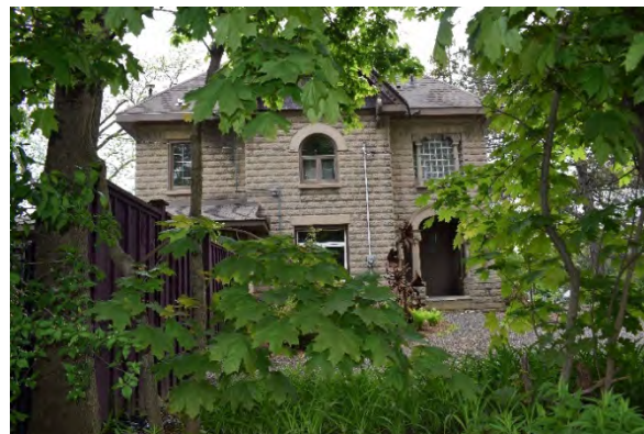
Plate 28: East façade of residence, looking west
