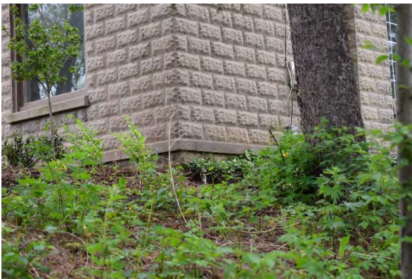
Plate 21: Concrete band between foundation blocks and exterior blocks, looking east
