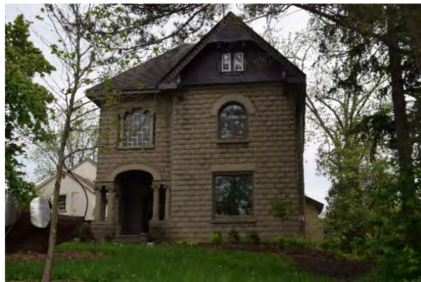
Plate 22: North façade, looking south
