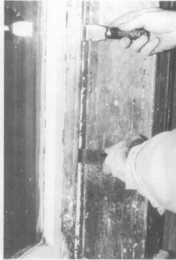
Figure 4b. After removing paint from the seam between the interior stop and the jamb, the stop can be pried out and gradually worked loose using a pair of putty knives as shown. To avoid visible scarring of the wood, the sash can be raised and the stop pried loose initially from the outer side. Photo: John H. Myers
