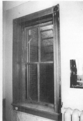
Figure 4f. Following the relatively simple repairs, the window is weathertight, like new in appearance, and serviceable for many years to come. Both the historic material and the detailing and craftsmanship of this original window have been preserved. Photo: John H. Myers
