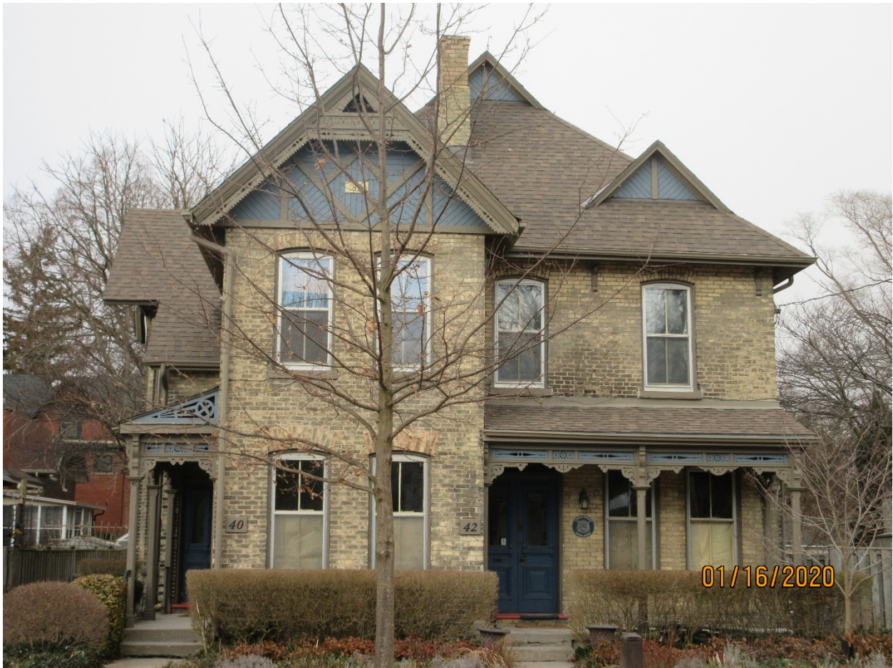
Image 3: Photograph of the properties at 40 & 42 Askin Street on January 16, 2020.
