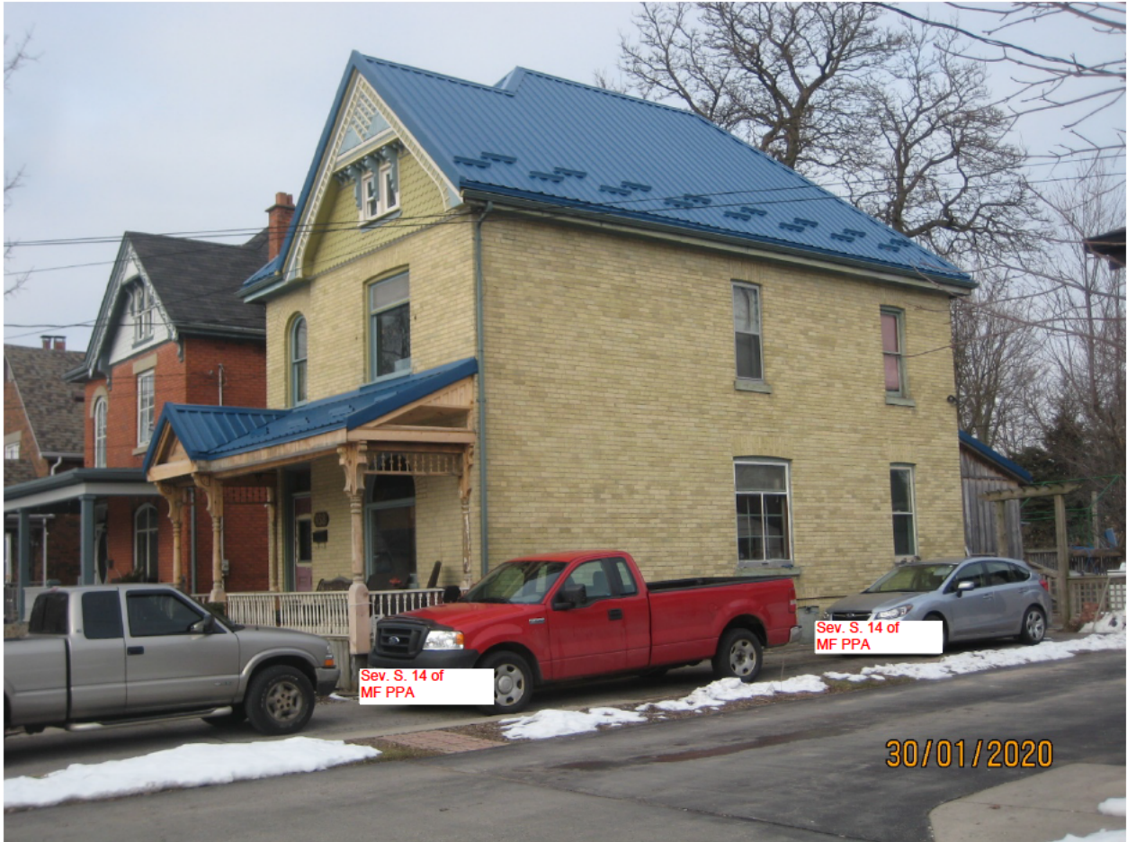
Image 11: Photograph showing the unapproved roof materials alterations completed, and existing status of porch in January 2020
