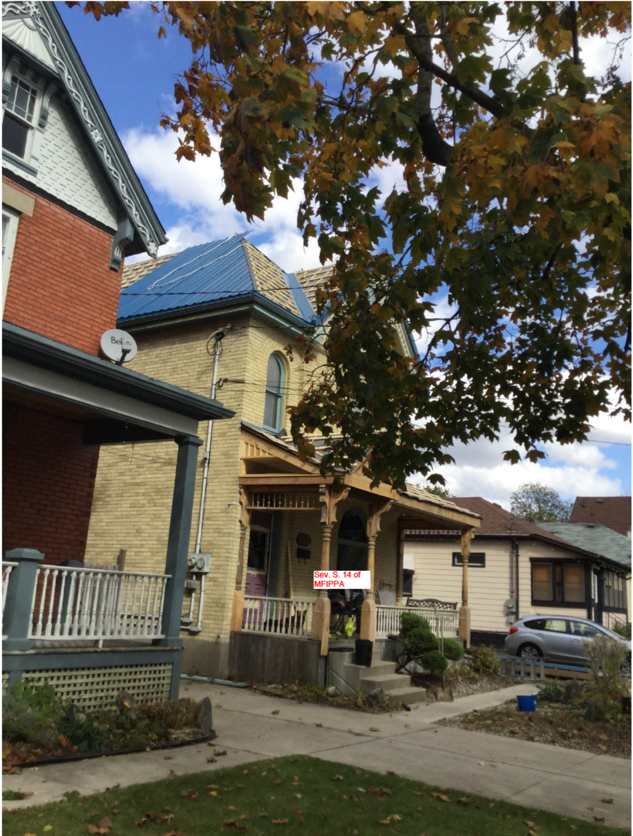
Image 5: Photograph submitted as a part of the Heritage Alteration Permit application showing unapproved alterations underway in October 2019
