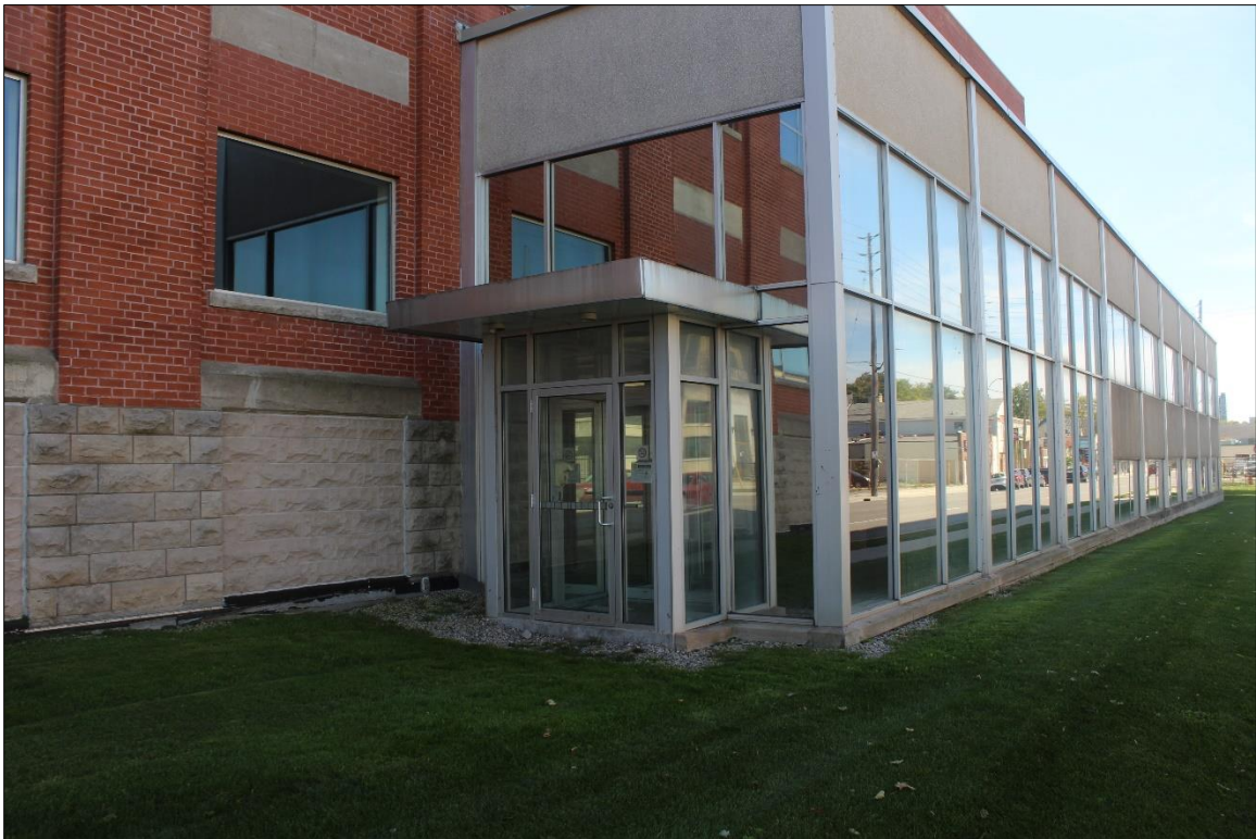
Image 7: 1960-61 glass and aluminium entranceway, north facade (AECOM, 2019)
