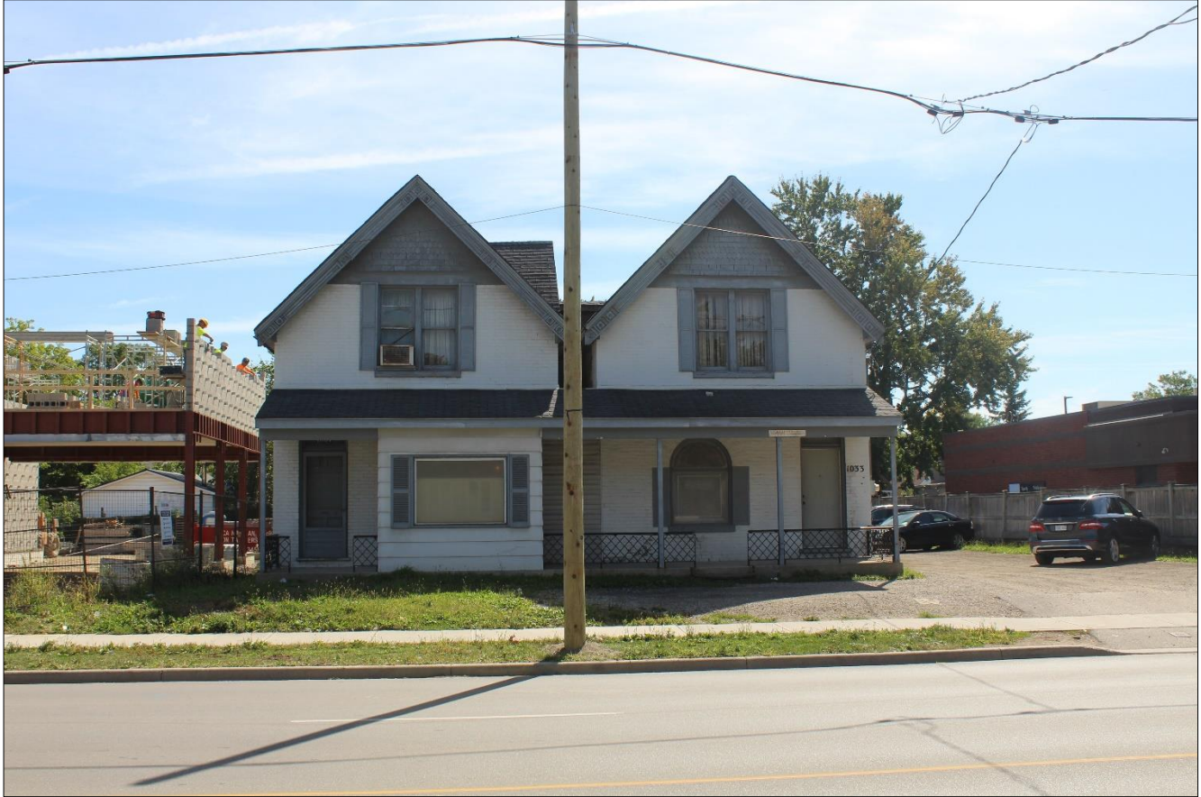
Image 1: Property at 1037 (left) and 1033 Dundas Street (right) (AECOM, 2019)
