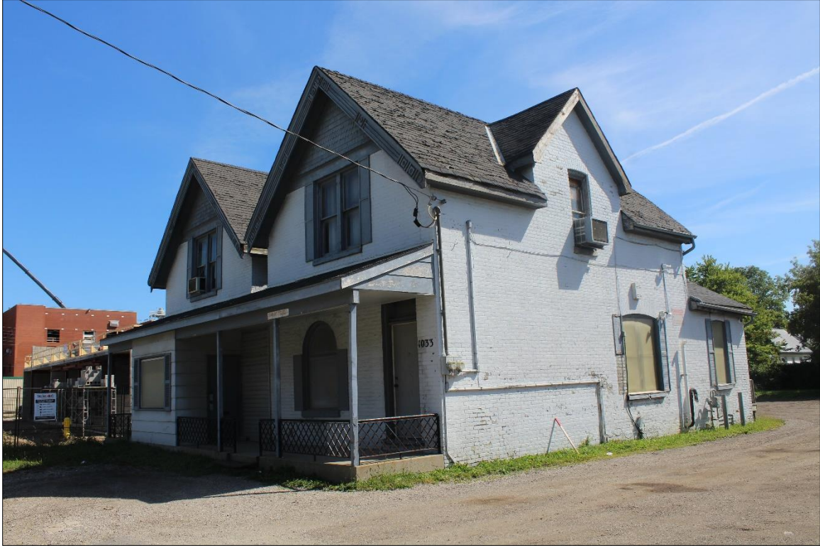
Image 2: Front (north) and west façades, 1033-1037 Dundas Street (AECOM, 2019)
