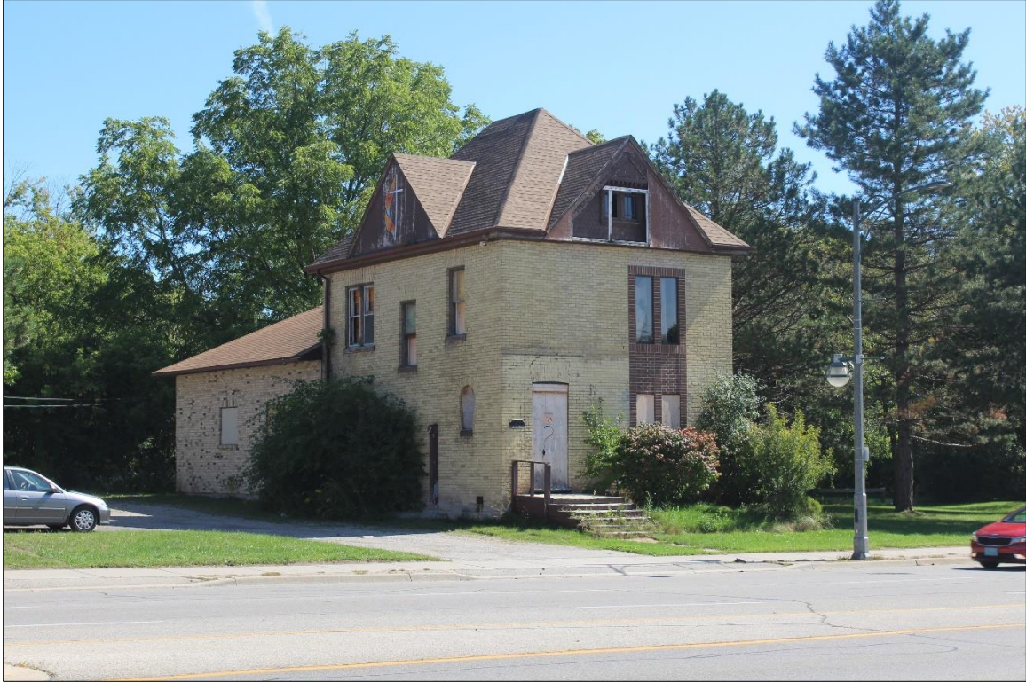
Image 2: Front (west) and north façades, 72 Wellington Street (AECOM, 2019)
