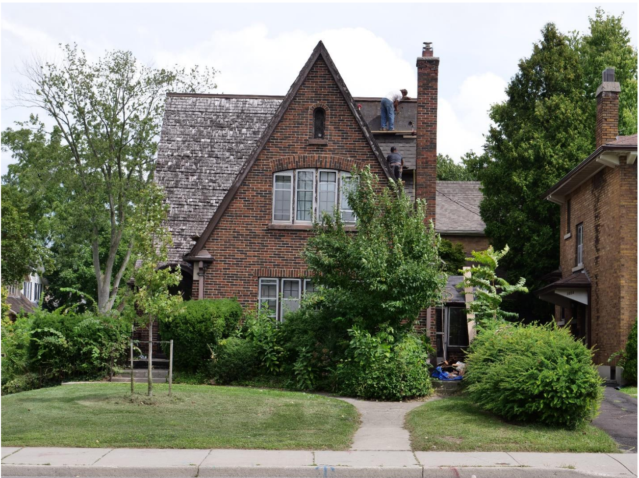
Image 4: Photograph of the property (front/west elevation) at 1058 Richmond Street on August 26, 2019 showing work underway to remove the wood shingle roof and replace it with asphalt shingles.
