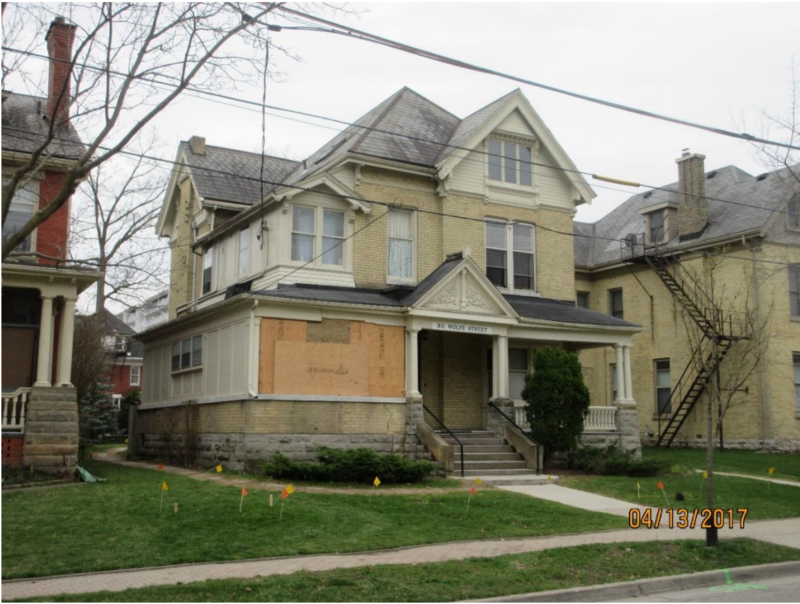
Image 14: Photograph of the property at 309-311 Wolfe Street, showing the original slate roof on April 13, 2017.
