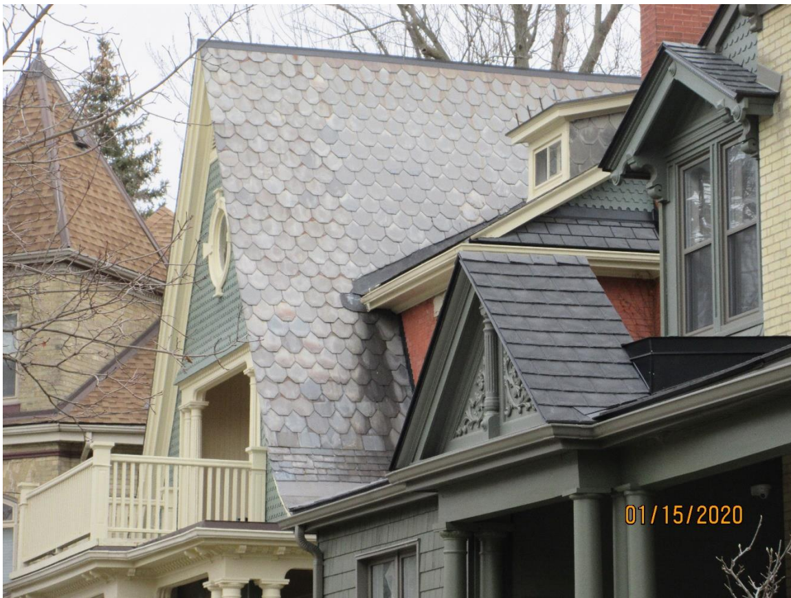
Image 16: Detail photograph showing the rubber composite product on the property at 309-311 Wolfe Street on January 15, 2020 contrasted with the slate shingles of the adjacent property at 315 Wolfe Street.
