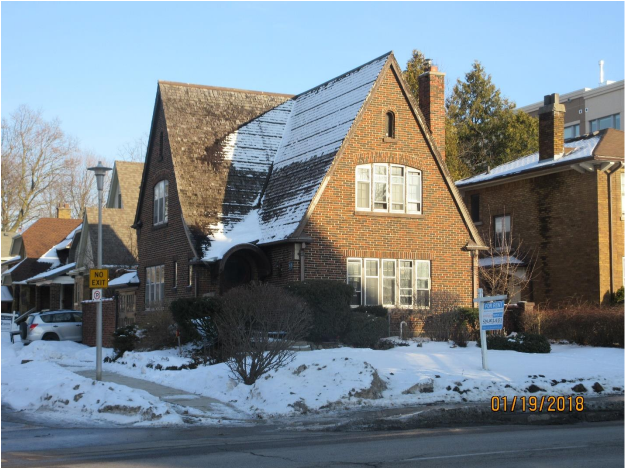
Image 3: Photograph of the property at 1058 Richmond Street (January 18, 2018).
