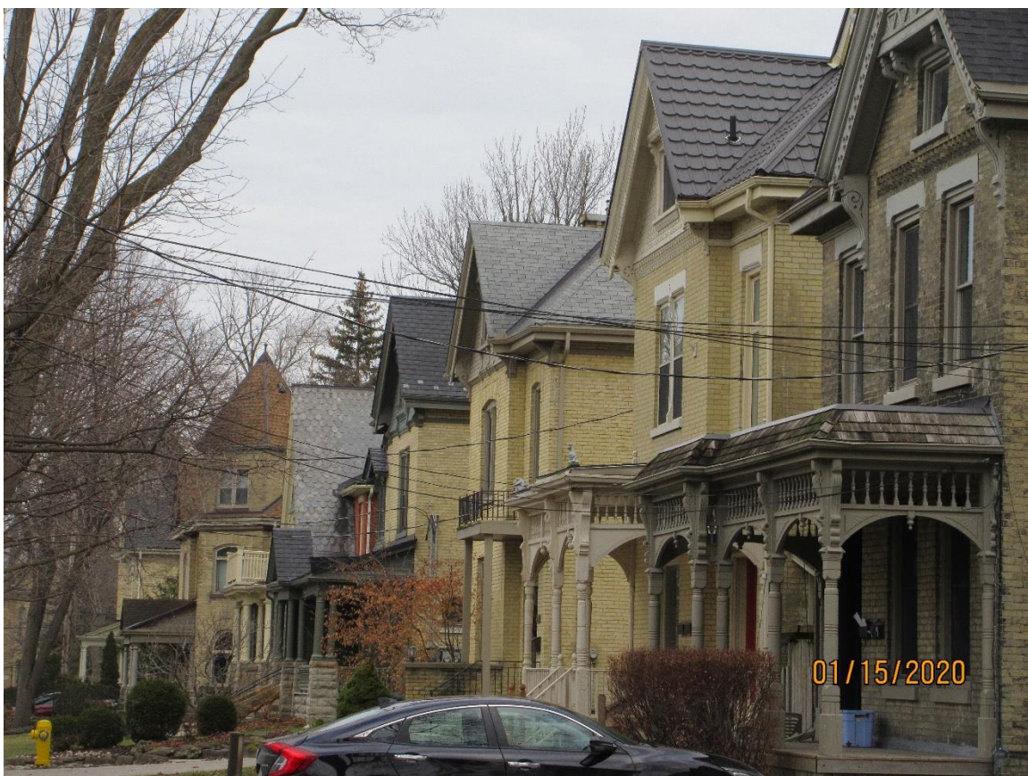
Image 17: Showing the streetscape of the south side of Wolfe Street, a variety of roofing materials can be seen. From right to left: asphalt shingles, metal roof, asphalt shingles, composite shingles, slate, and asphalt shingles. Some roofing materials are clearly more compatible with the heritage character of the West Woodfield Heritage Conservation District and the individual cultural heritage resources.
