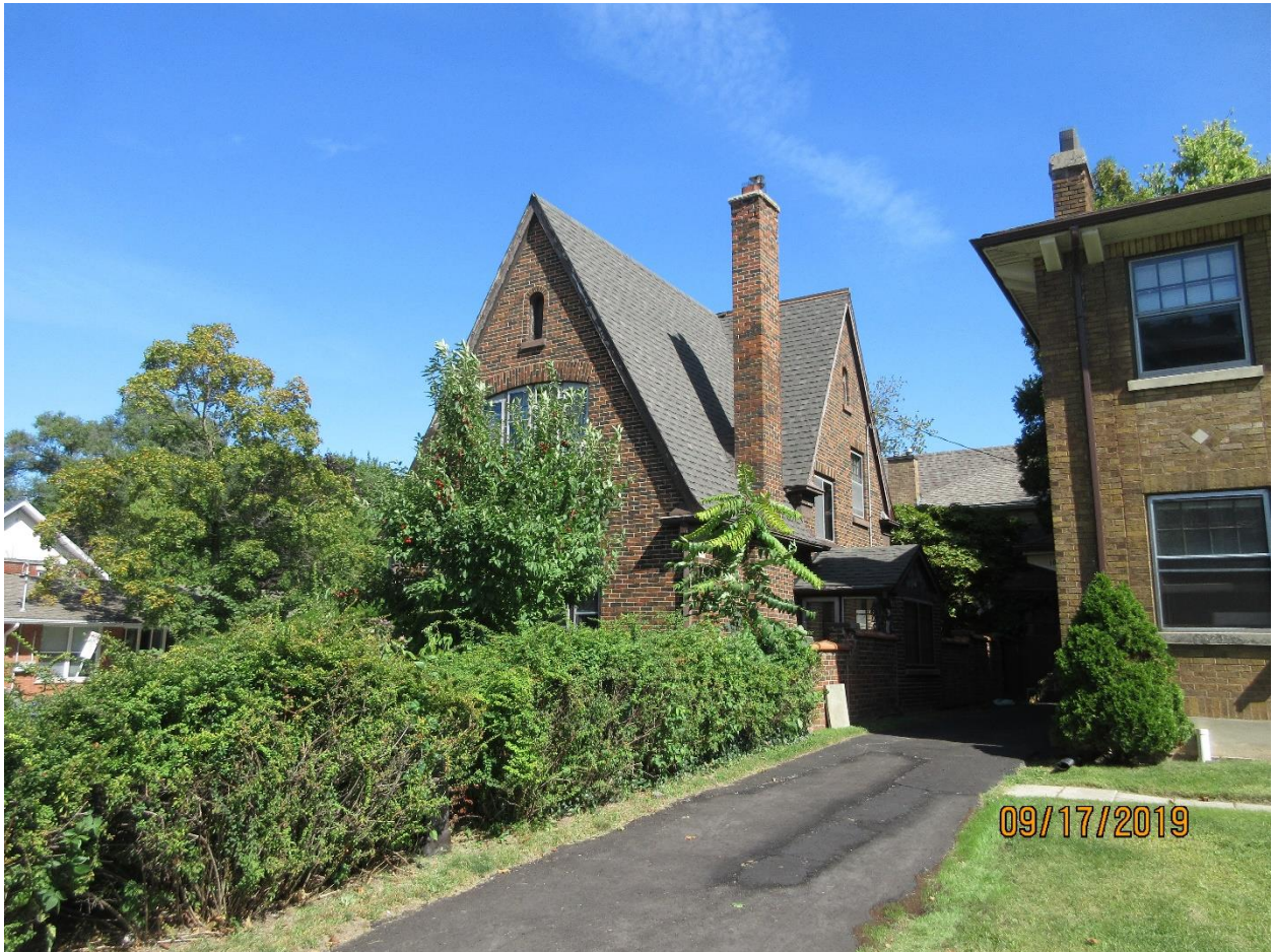
Image 11: Photograph showing the completed roofing replacement with asphalt shingles on the property at 1058 Richmond Street (front/west and south elevations) on September 17, 2019.
