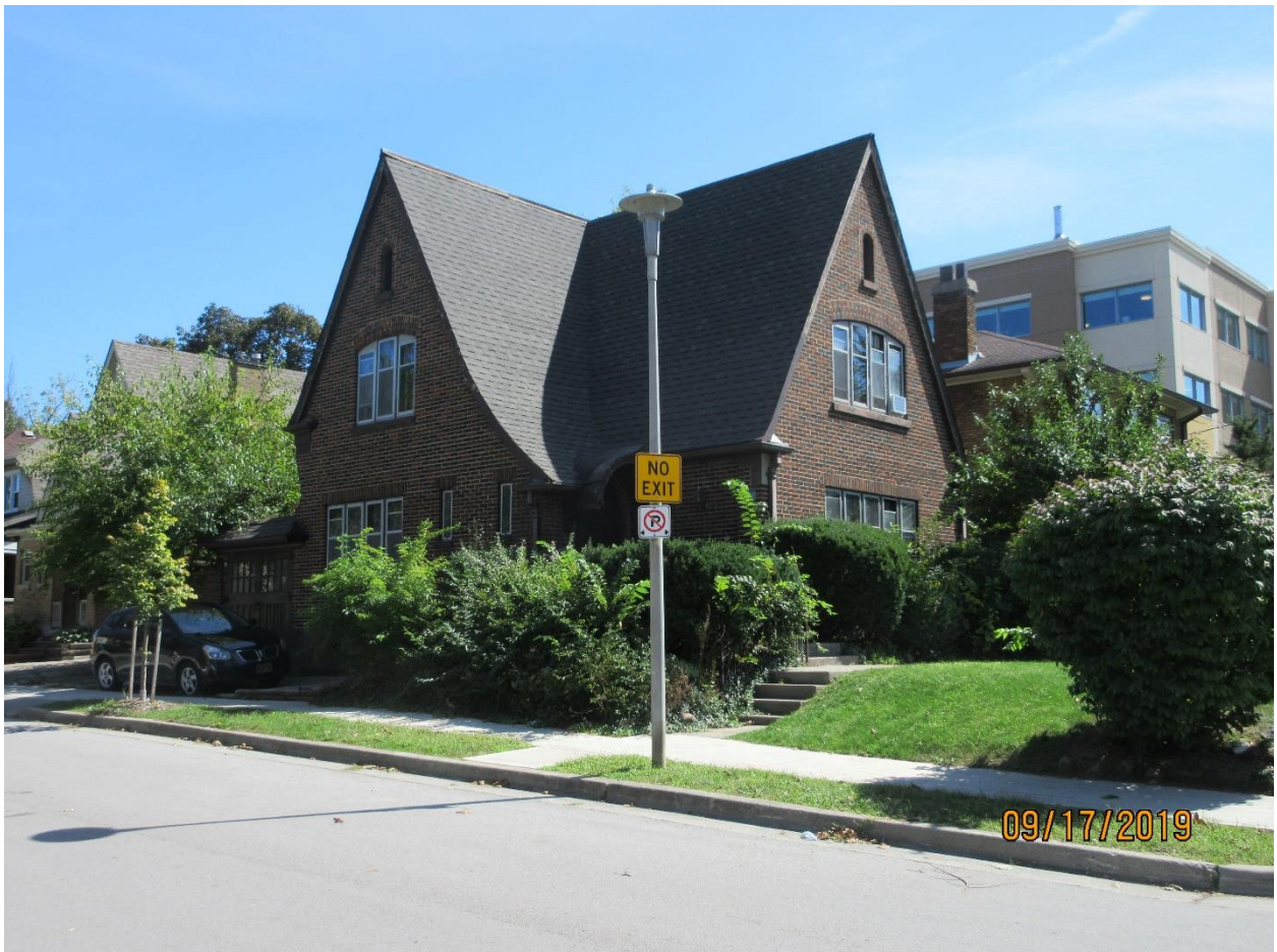
Image 8: Photograph showing the completed roofing replacement with asphalt shingles on the property at 1058 Richmond Street (north and front/west elevations) on September 17, 2019.
