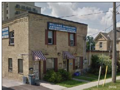
Apart from a new door in the centre, the main Kent Brewery building (left) and its washhouse (right) still look much as they did in their heyday, when the c. 1905 photograph was taken. The building is currently the Williams Downtown Automotive Service at 197 Ann Street. The building today is the "largest surviving brewery artifact from Victorian London Middlesex". (Phillips, 155). The Brewery was already considered old in the 19th Century. In 1889, Goodspeed's History of the County of Middlesex said of the Kent Brewery: "The premises form one of the oldest landmarks in the city, and are located on Ann Street." (Goodspeed, p. 373)
