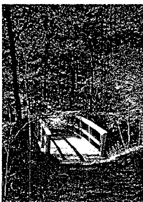
Wood and steel pedestrian bridge in Medway Valley Heritage Forest ESA
