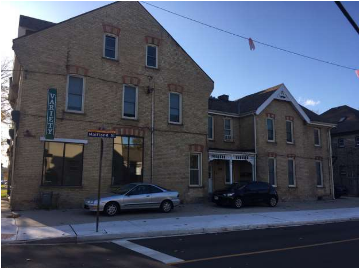
Figure 2: Subject site (view from Maitland Street)
