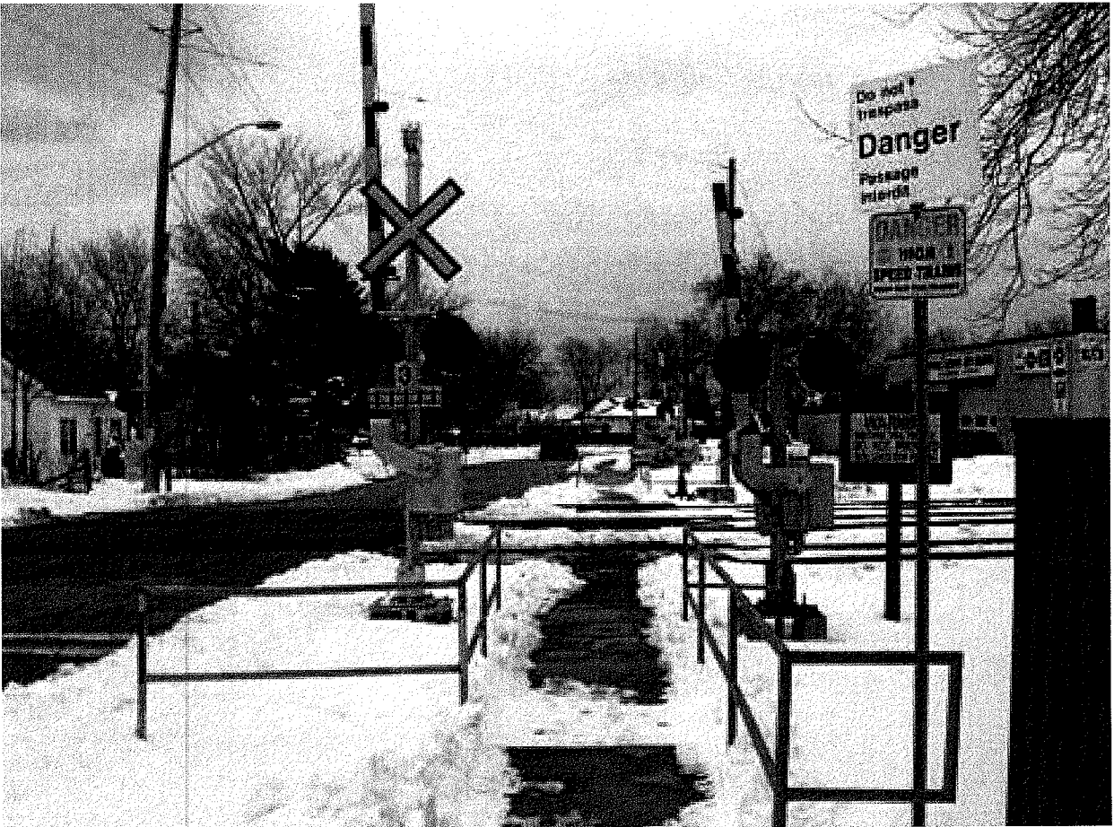
Figure 4 - Pedestrian gate installation
