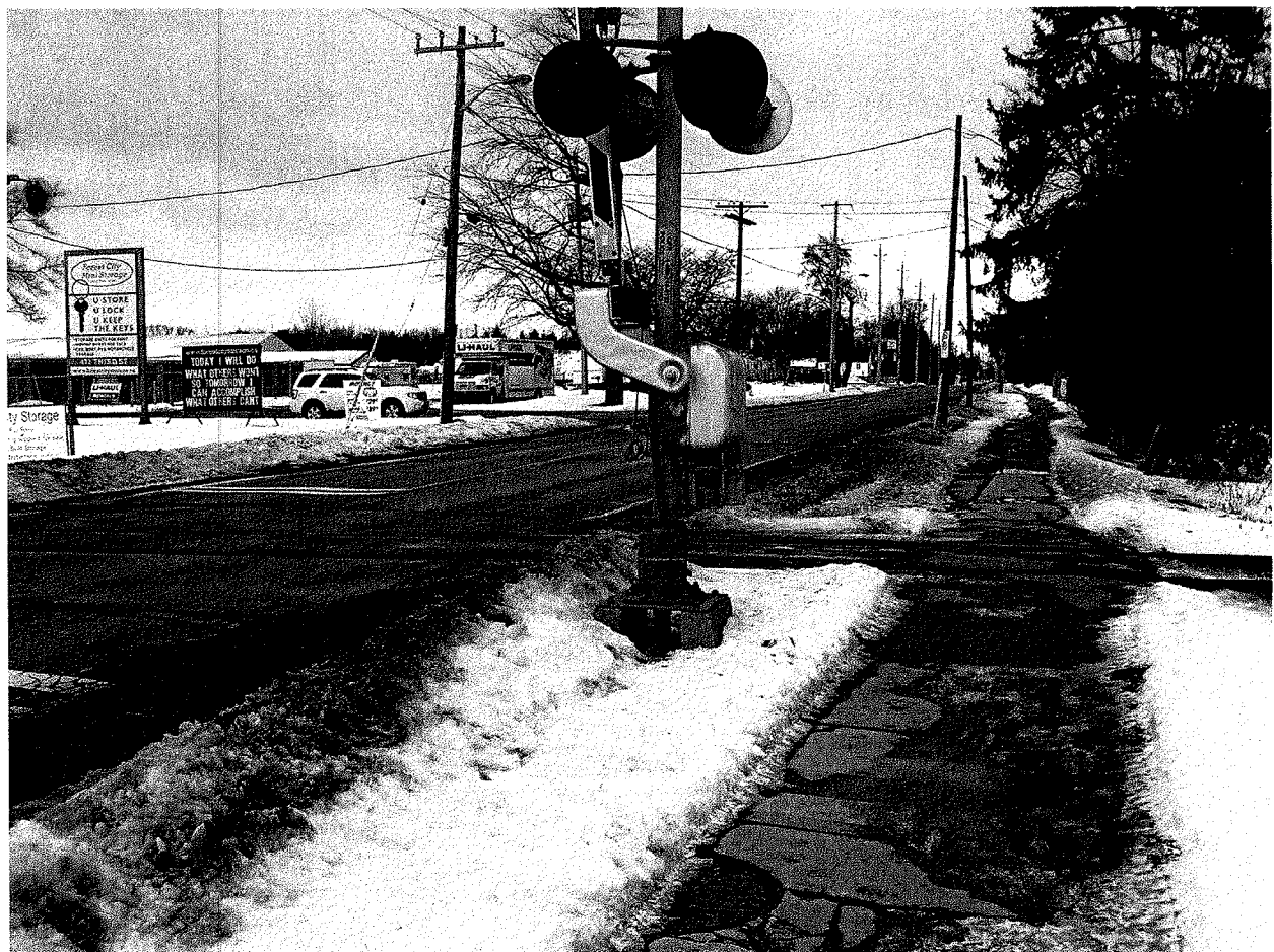
Figure 2 - Third Street sidewalk looking north
