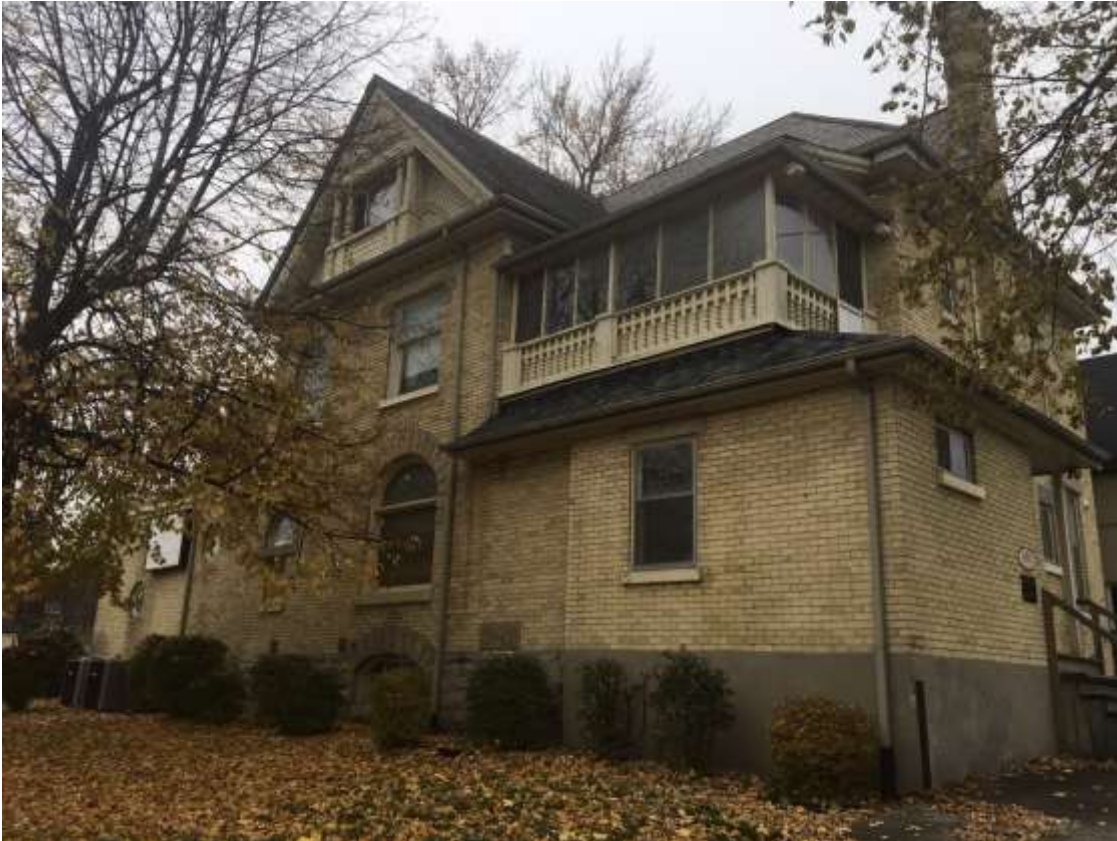
Figure 1: Subject site (view off of Central Avenue).
