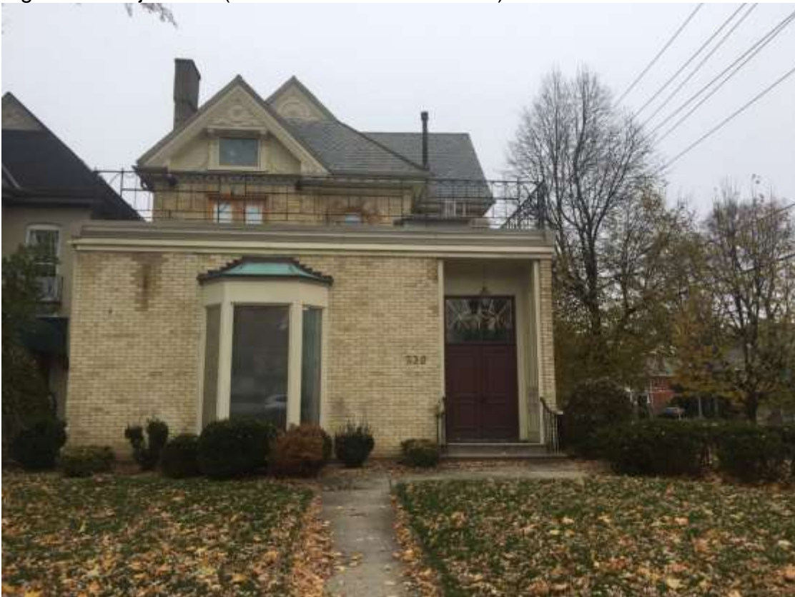
Figure 2: Subject site (view off of Waterloo Street).
