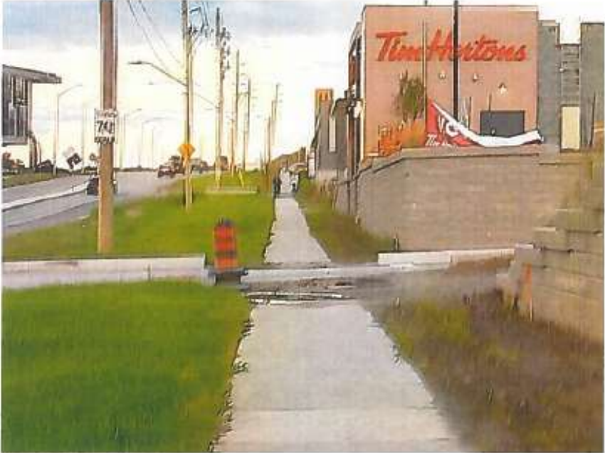
Image 5 – Driveways limiting direct access to Oxford Street to drive through restaurants, and median separating west bound traffic from entering the restaurants.
