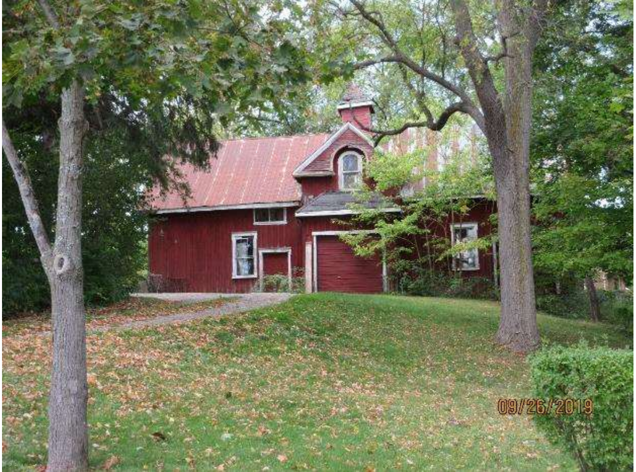
Image 10: Photograph showing the accessory building in September 2019
