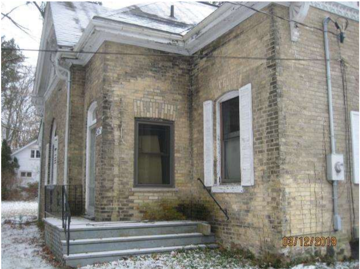
Image 16: Detail showing window/doorway alterations on the east elevation to 247 Halls Mill Road, December 2019.
