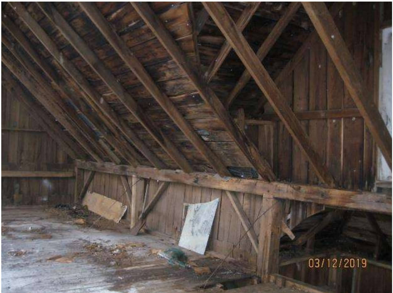
Image 28: Interior detail of the mortise and tenon timber frame construction and roof rafters on the east side of the accessory building, December 3, 2019.
