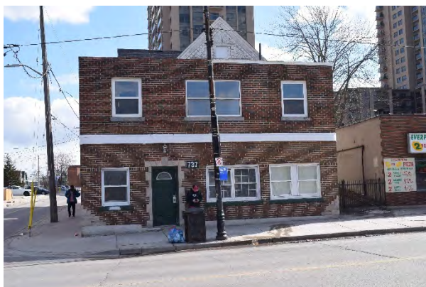
Plate 16: Front façade of northern addition, looking south
