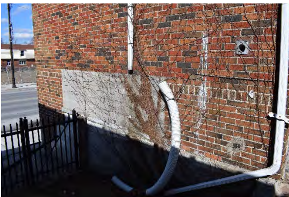
Plate 22: West façade of north addition, looking east
