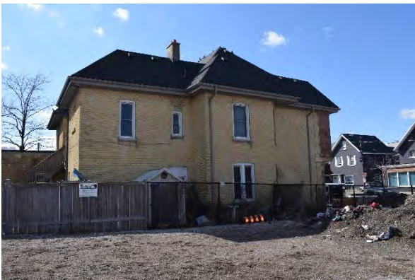
Plate 35: East façade, looking west
