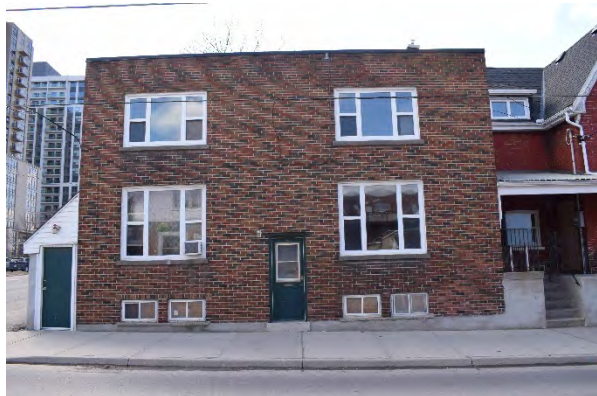
Plate 19: East façade of rear addition, looking west
