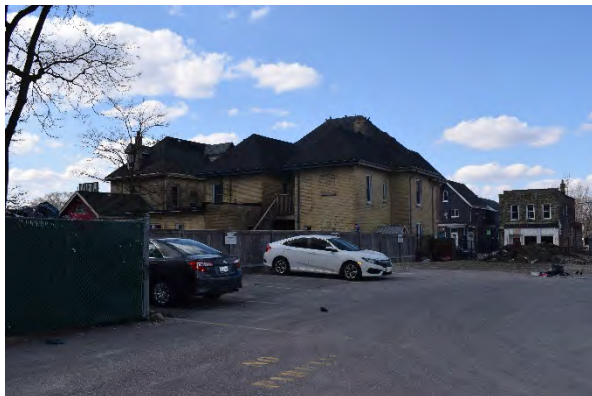
Plate 36: Rear (south) façade, looking north
