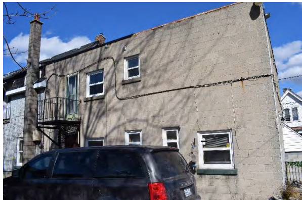
Plate 21: West façade of rear addition, looking east
