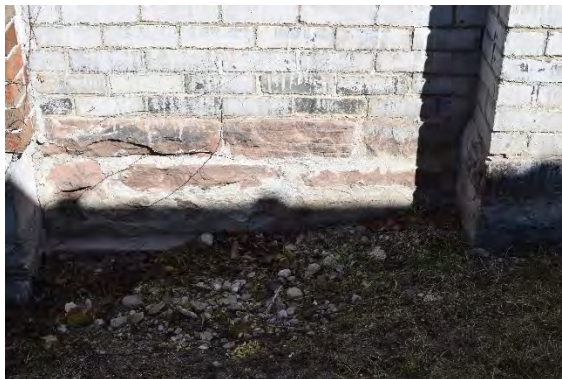
Plate 13: Rusticated concrete block foundation, looking east
