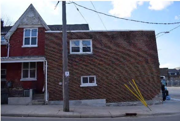
Plate 18: East façade of north addition, looking west
