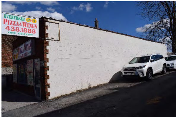
Plate 25: West façade of 735 Dundas Street, looking east
