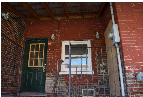
Plate 14: Replacement window and door openings, looking west
