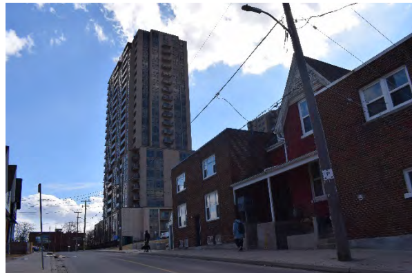
Plate 4: Revo high rise apartment building, looking south
