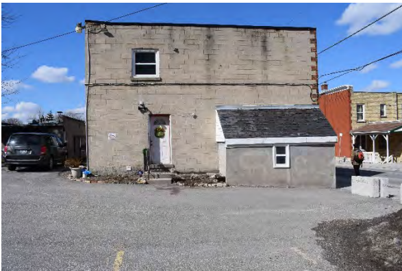
Plate 20: South façade, looking north
