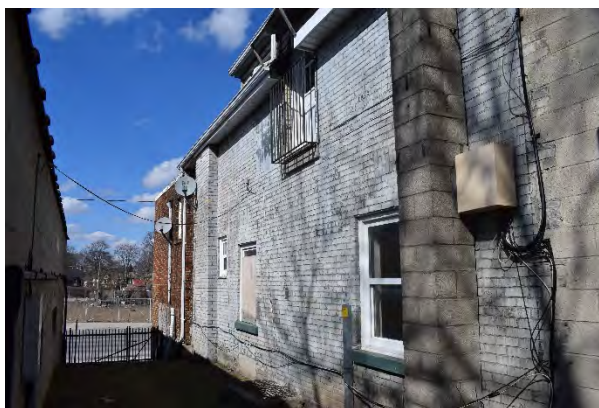
Plate 15: Original portion of west façade, looking north
