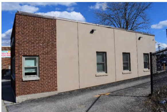
Plate 30: West façade of 729 Dundas Street, looking east
