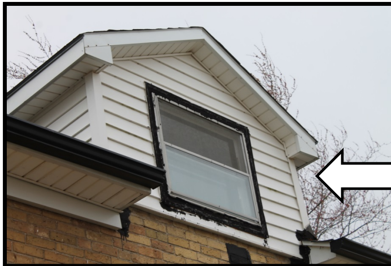
Shed dormer covered with siding. Original window replaced.
