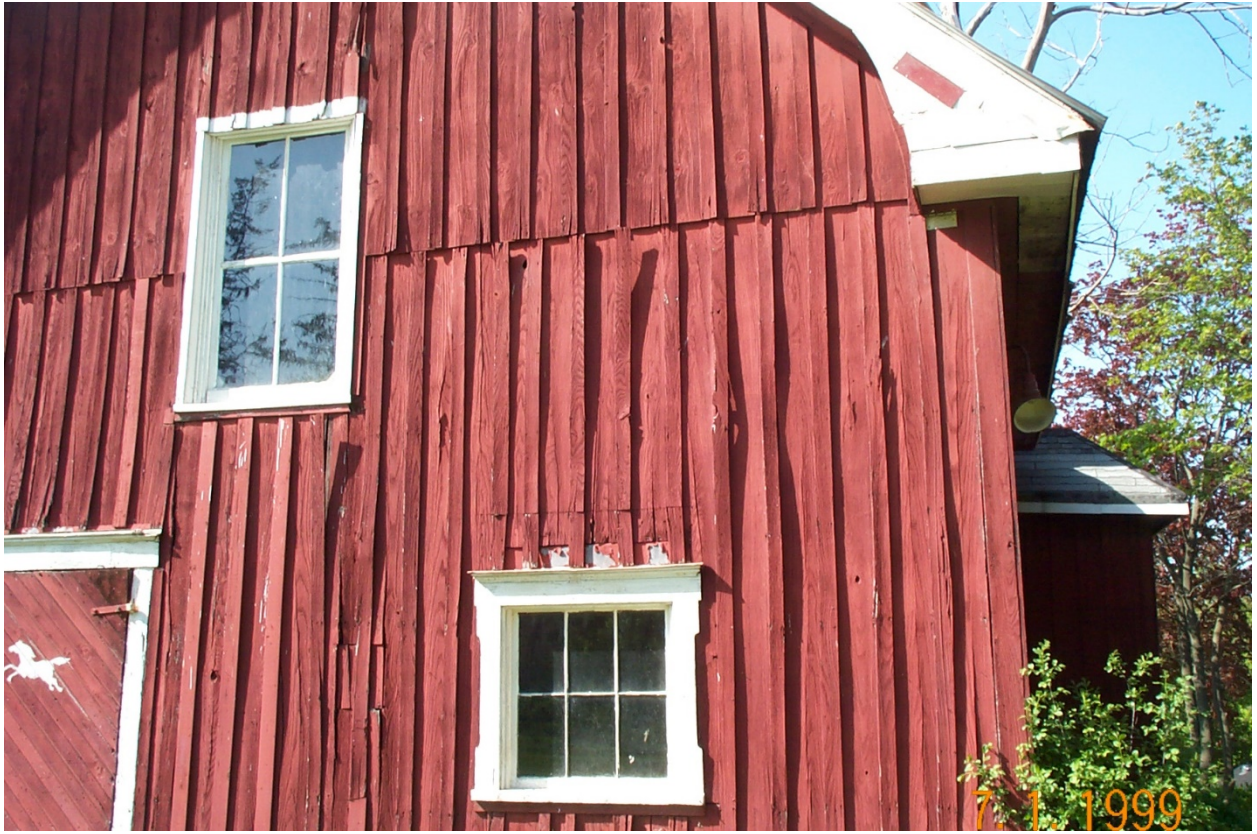
Image 9: Photograph of the south side of the accessory building, showing board and batten exterior cladding and window details, 1999.
