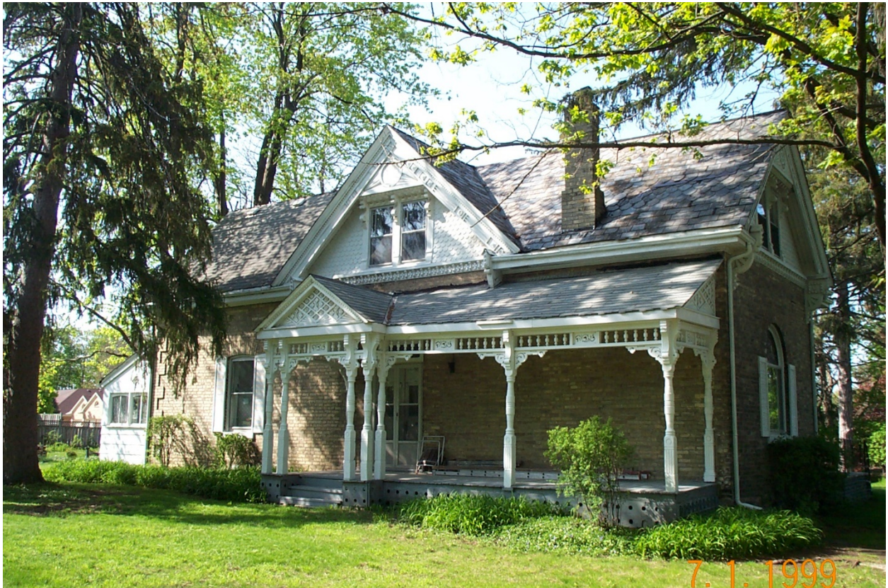
Image 2: Photograph of the south façade of the dwelling at 247 Halls Mill Road, 1999.
