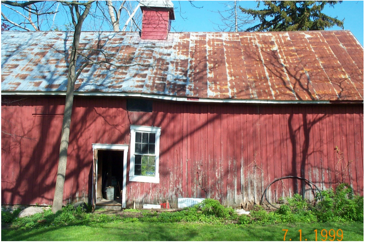
Image 7: Photograph of the west side of the accessory building, 1999.
