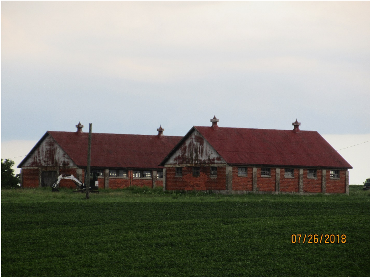
Image 39: Property at 660 Sunningdale Road East, part IV designated
