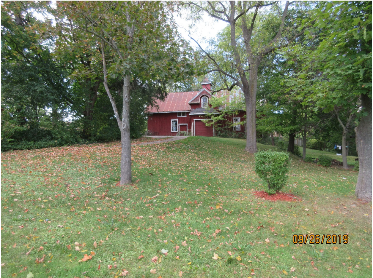
Image 11: Photograph of the accessory building as viewed from Halls Mill Road, September 2019.
