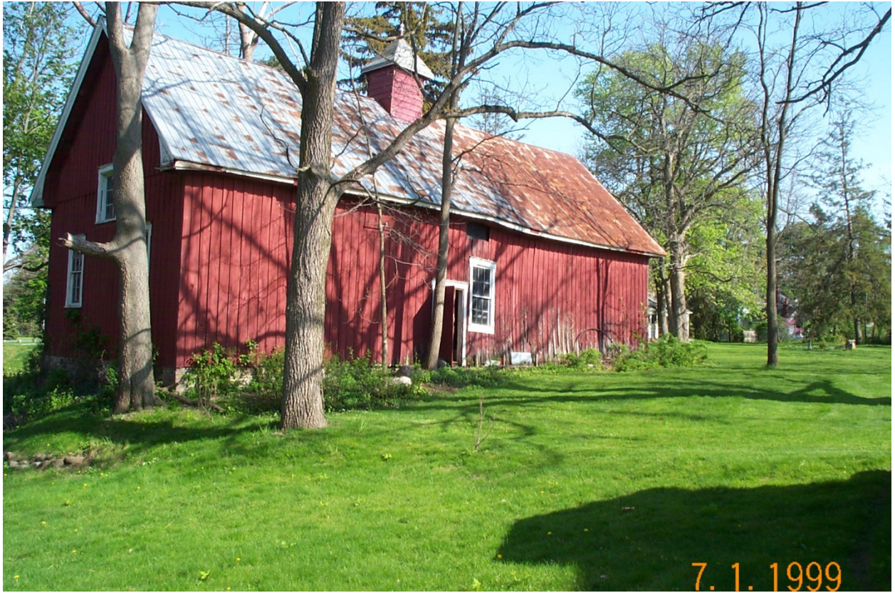
Image 6: Photograph of the west side of the accessory building, 1999.
