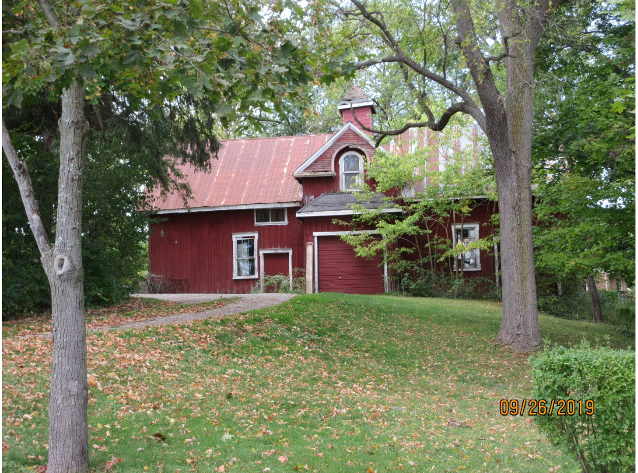
Image 10: Photograph showing the accessory building in September 2019
