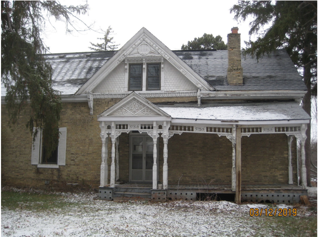
Image 17: Photograph showing the south elevation of the dwelling at 247 Halls Mill Road, showing decorative elements and south porch
