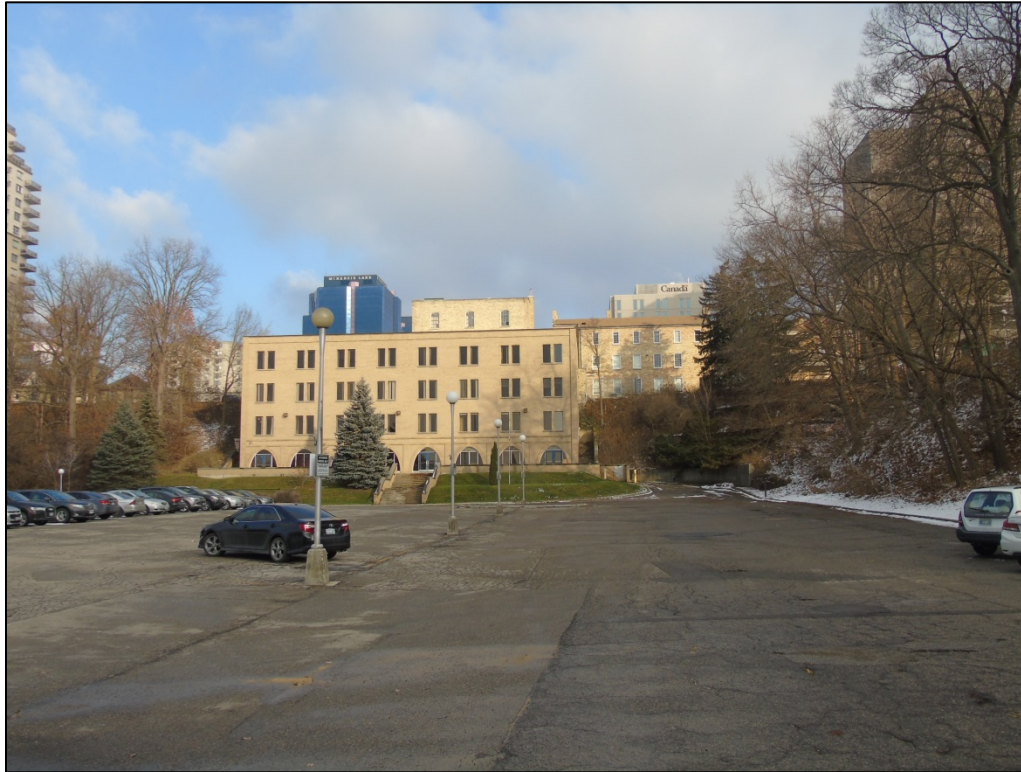
Image 7: View showing modern commercial structure constructed to the rear of 451 Ridout Street North, built into the embankment
