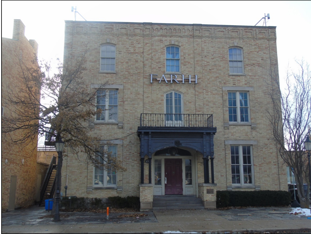
Image 3: View showing heritage building at 451 Ridout Street North
