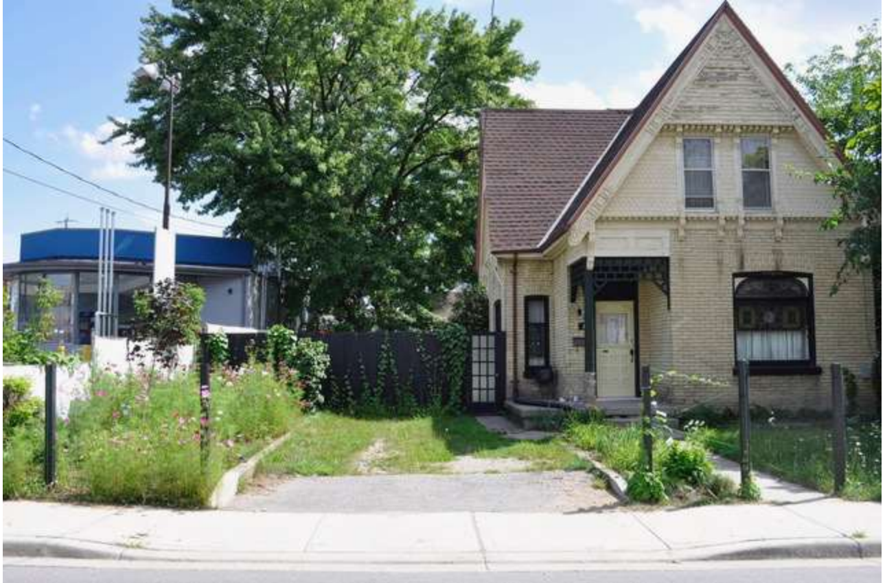
Fig. 10 : Vent pipe location shown in relation to my doors and windows. Two doors and five windows face north. Four windows face west, as does the front door
