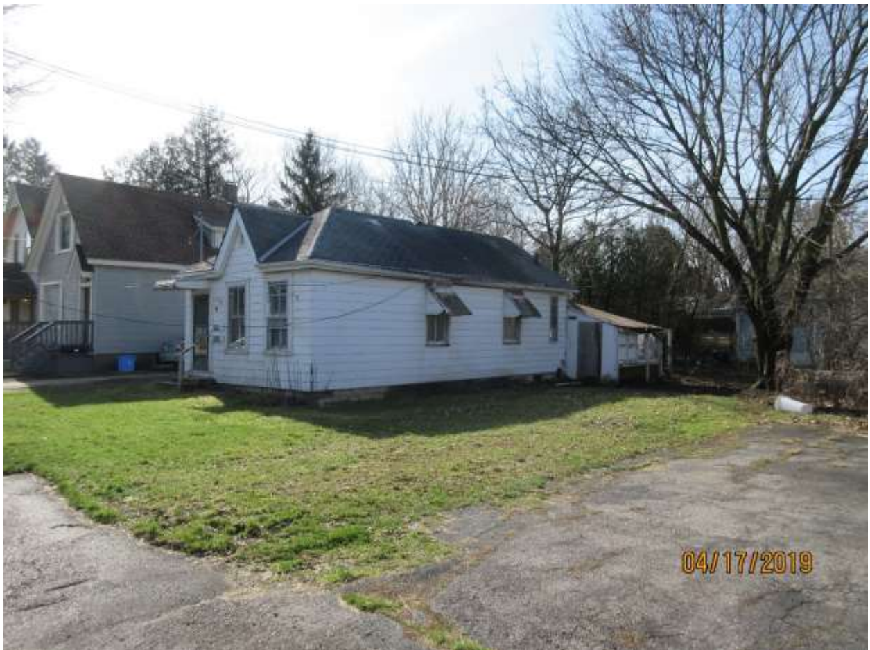
Image 4: View of the main (north) and west elevations of the Contributing Resource at 88 Blackfriars Street on April 17, 2019.
