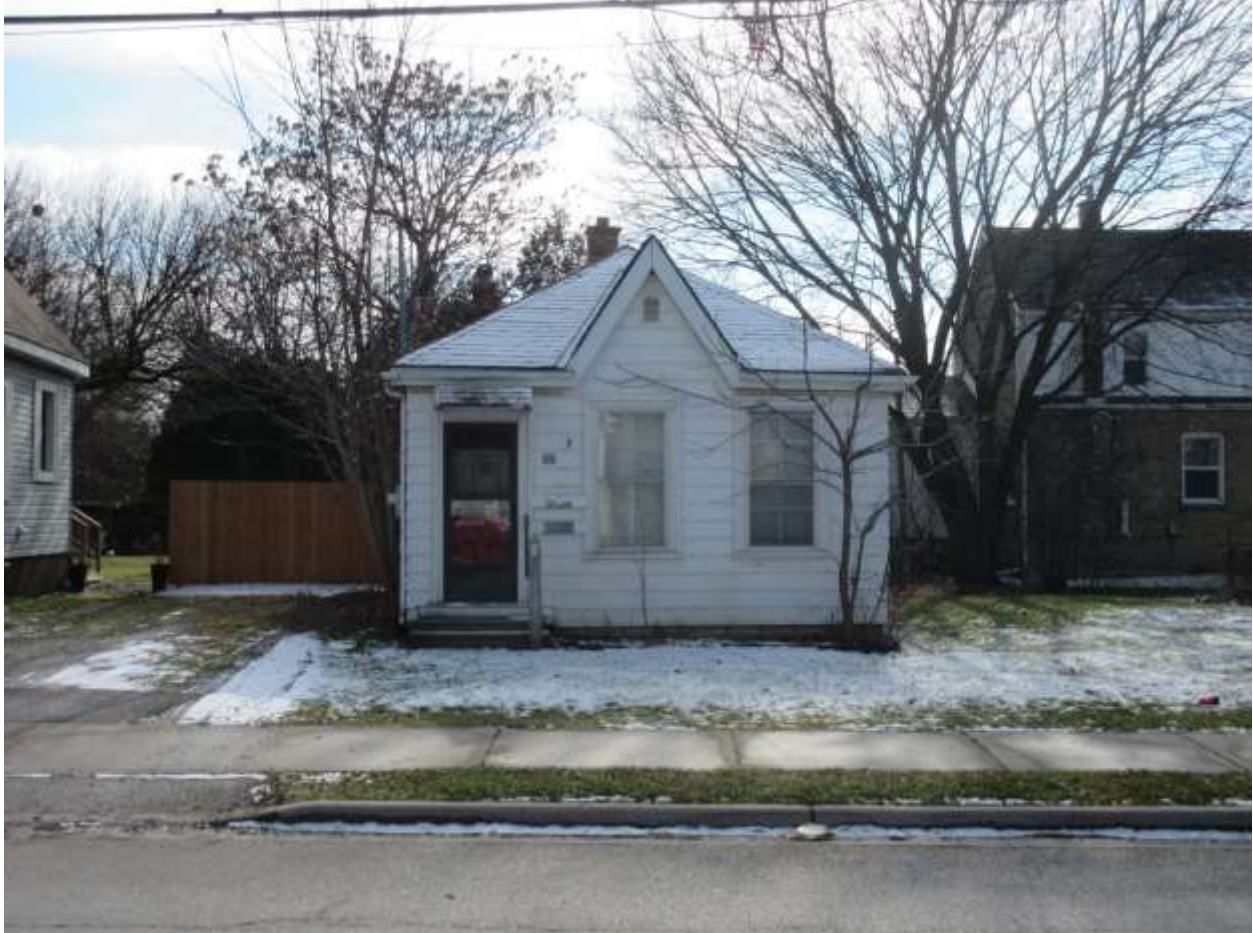
Image 1: The Contributing Resource at 88 Blackfriars Street on February 5, 2016.
