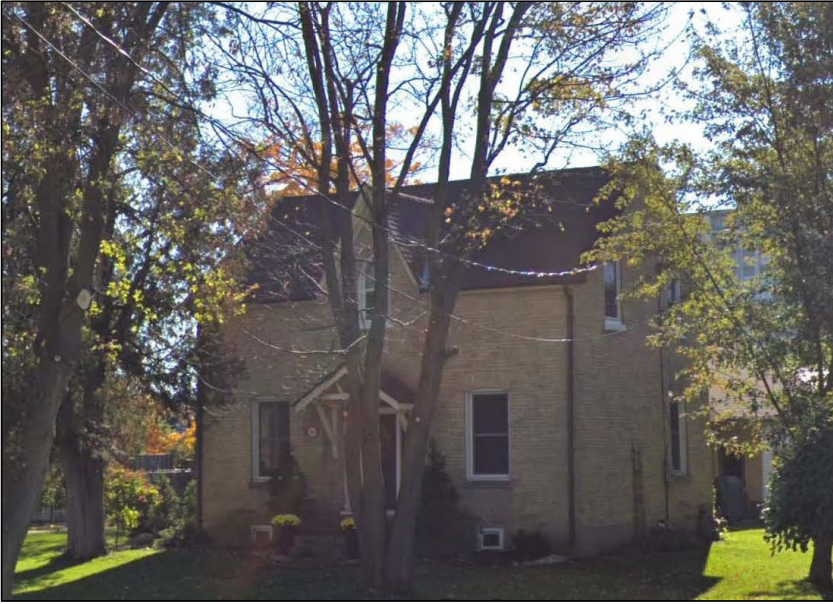
1006 Gainsborough Road - Current
