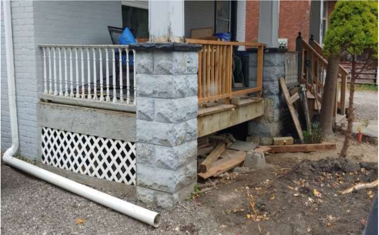
Image 5: Photograph showing the unapproved alterations underway at 906 Lorne Avenue submitted as a part of the Heritage Alteration Permit application. The existing railing and square spindles are shown on the left, and the proposed replacement railings are shown on the right of the post (October 2019). Note, a new lattice porch skirt and base of the column should be added as a part of the Heritage Alteration Permit.
