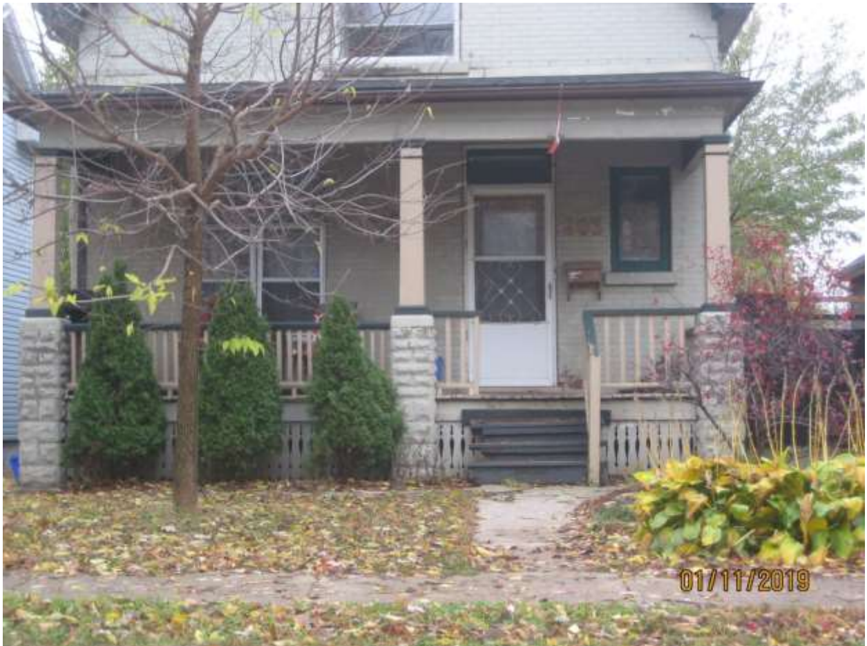
Image 7: Photograph of 903 Dufferin Avenue, also included within the Old East Heritage Conservation District, showing a railing and squared spindle design that is similar to the proposed design for 906 Lorne Avenue. Note, the heights of the top rails have also been raised on this porch, similar to the proposed design for 906 Lorne Avenue.
