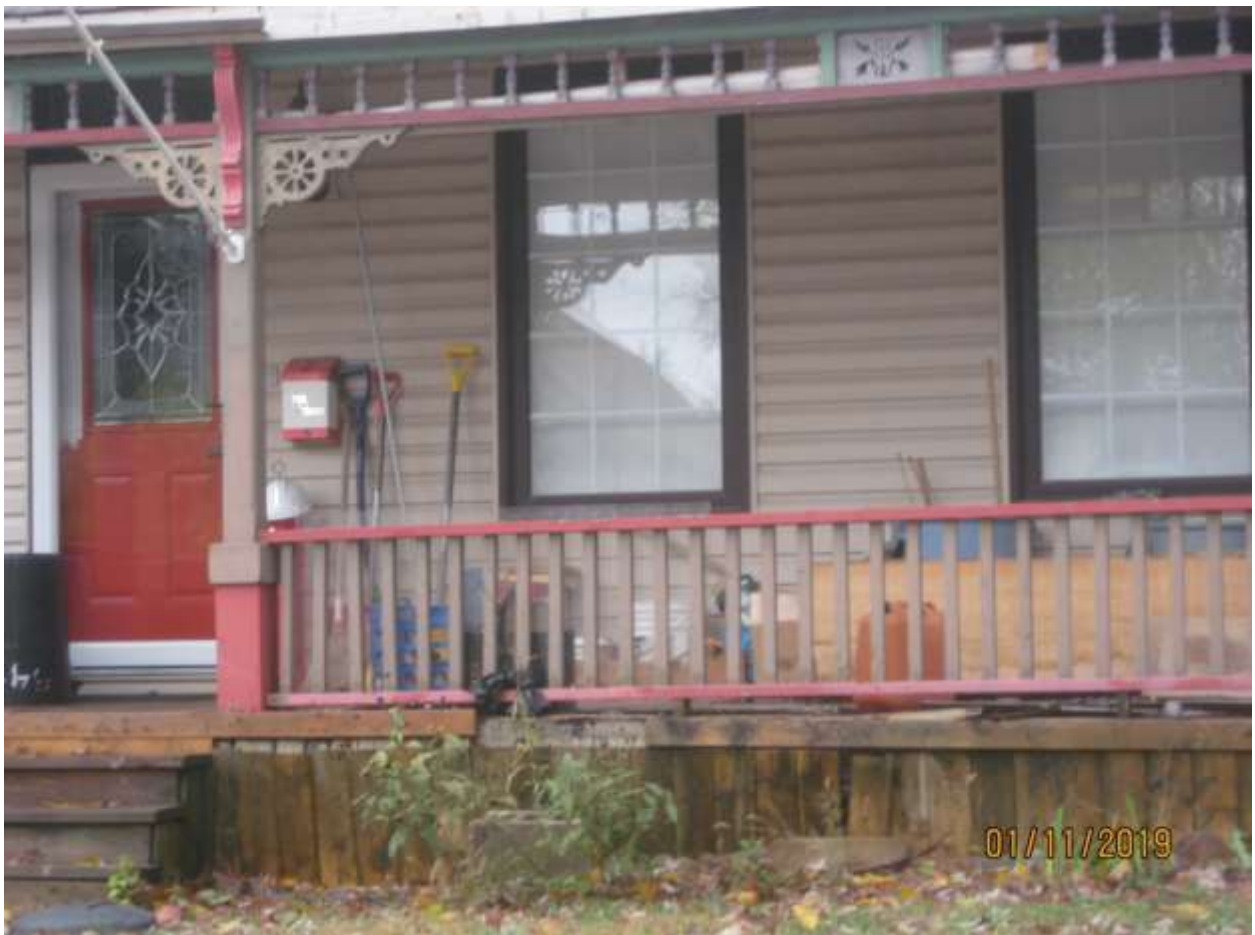
Image 8: Photograph of 944 Dufferin Avenue, also included within the Old East Heritage Conservation District, showing a railing and squared spindle design that is similar to the proposed for 906 Lorne Avenue. Although the trimwork on this verandah includes decorative turned millwork, the railing and spindles are squared, similar to the proposed design for 906 Lorne Avenue.
