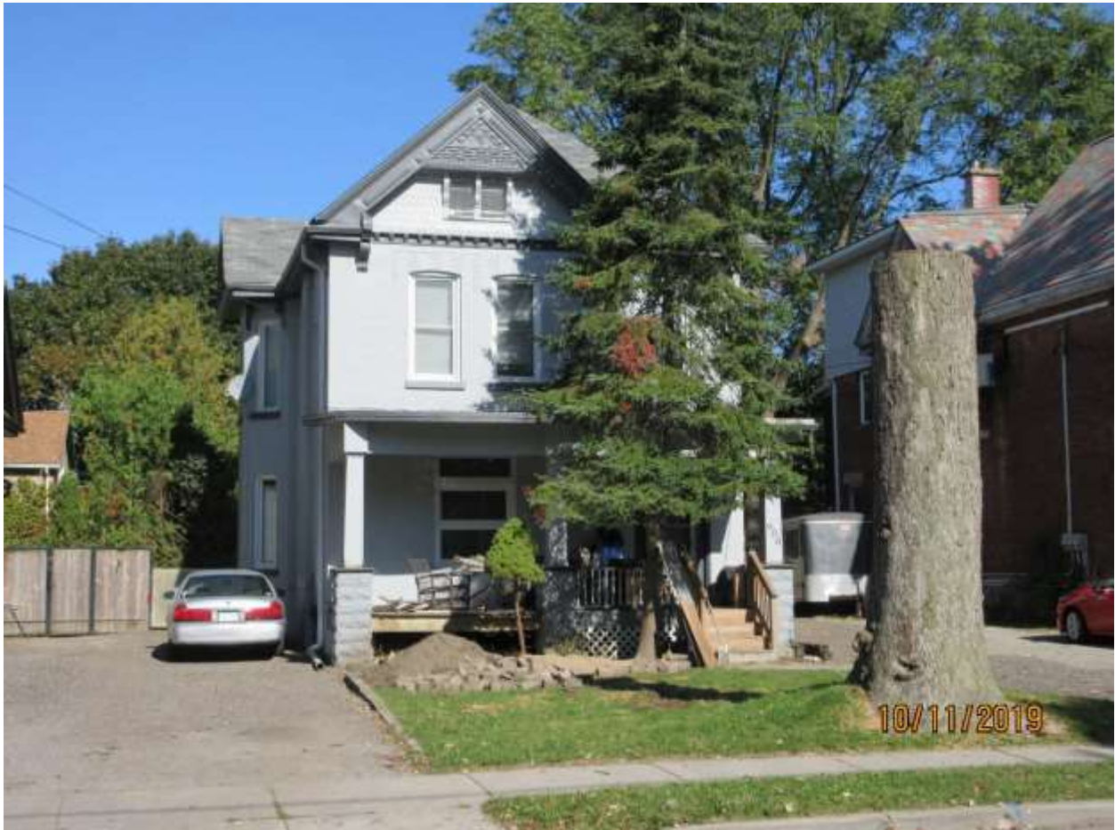
Image 1: Photograph of the property at 906 Lorne Avenue showing unapproved alterations underway, photographed on October 11, 2019.
