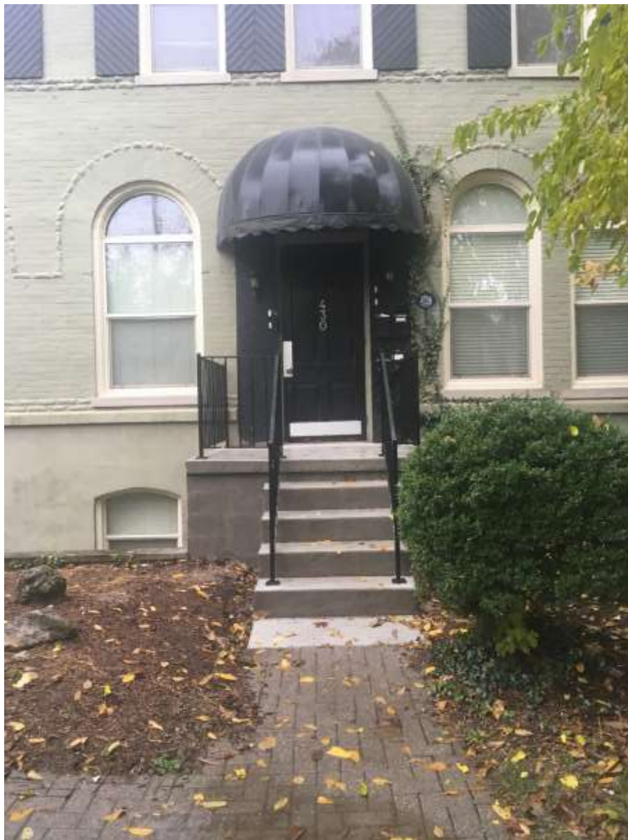
Image 6: Photograph showing the completed alterations to the porch, including re-pouring the concrete and new railings, of the property at 430 Dufferin Avenue (submitted as part of the Heritage Alteration Permit application).
