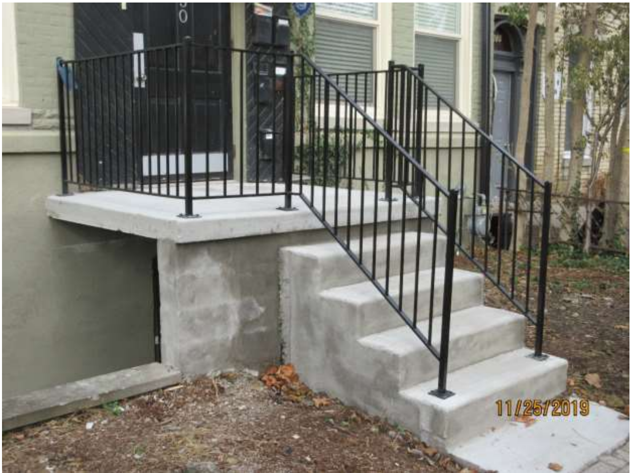
Image 8: Detail photograph of the new front porch on the property at 430 Dufferin Avenue.
