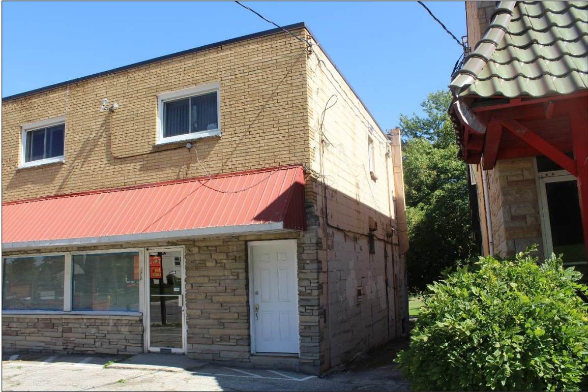
Image 2: Detail of south facade (AECOM, 2019)
