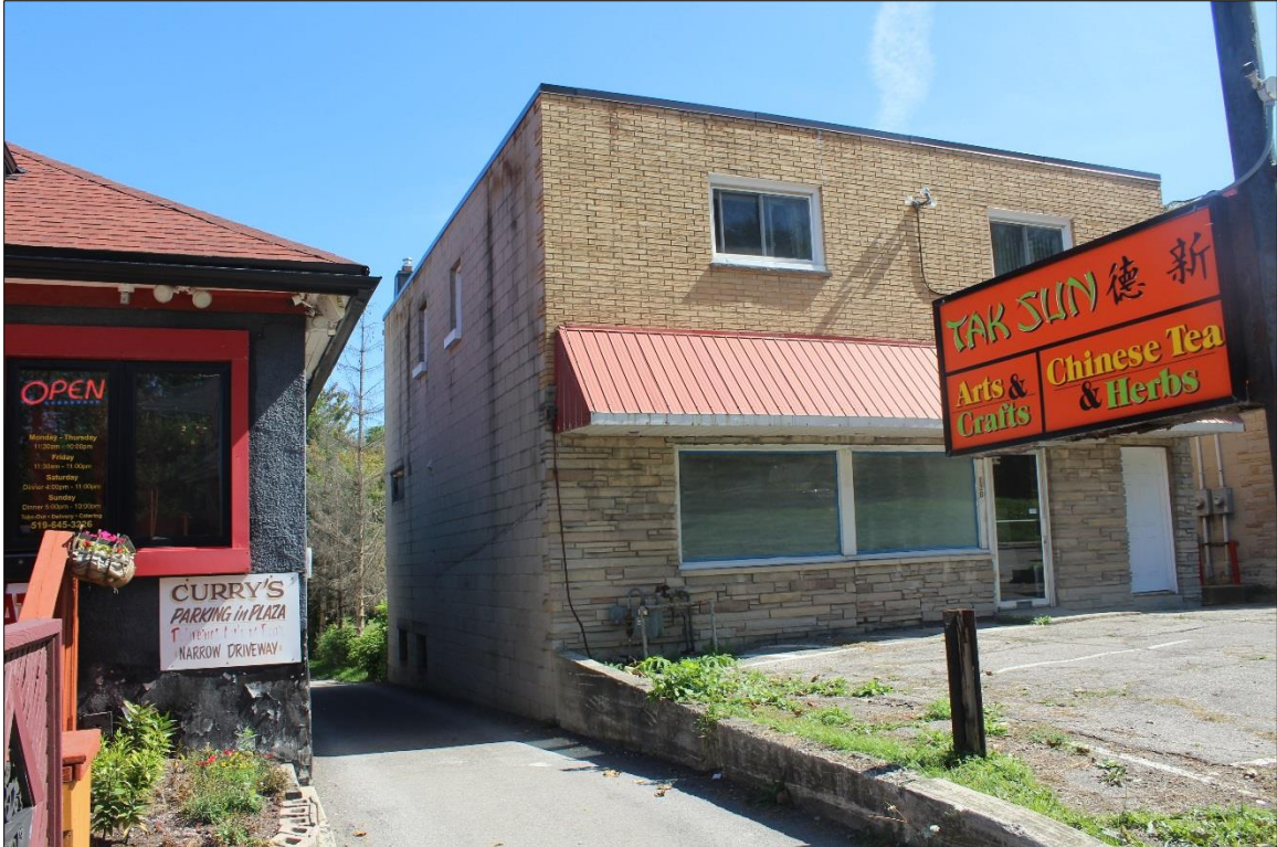
Image 3: Detail of north facade (AECOM, 2019)
