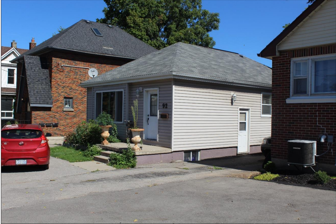
Image 2: South facade (AECOM, 2019)
