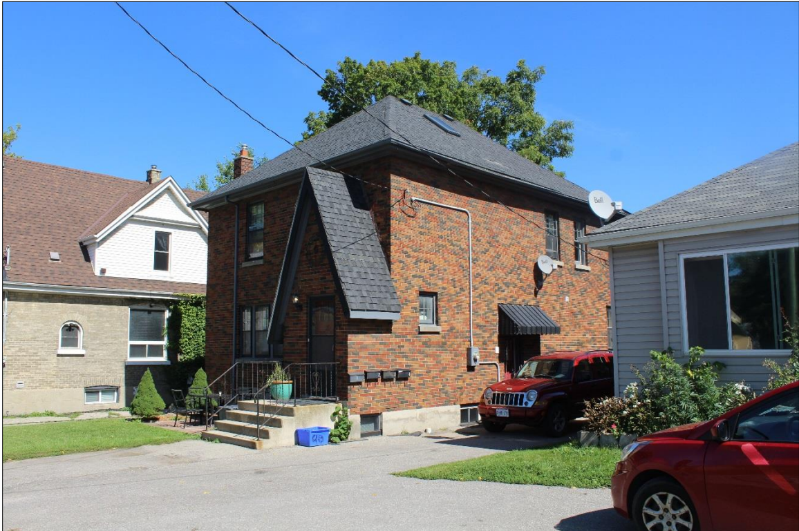
Image 3: South façade of 90 Wellington Road (AECOM, 2019)
