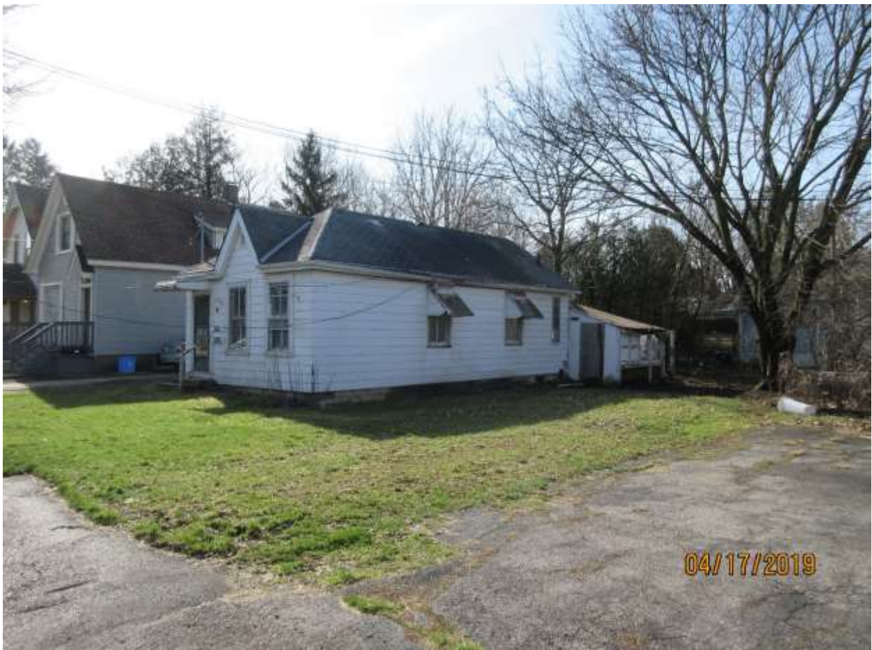
Image 4: View of the main (north) and west elevations of the Contributing Resource at 88 Blackfriars Street on April 17, 2019.
