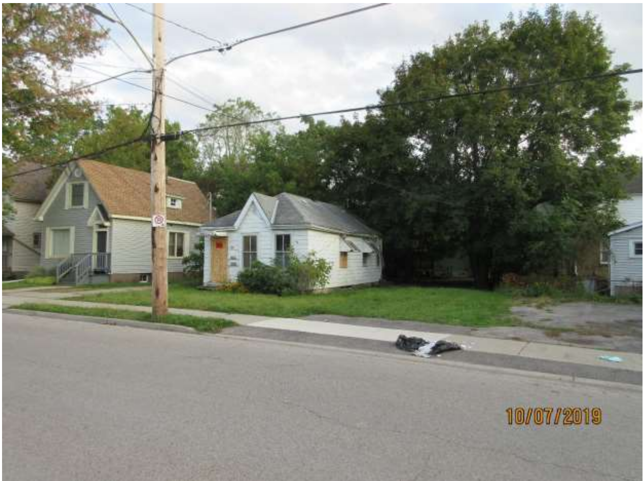
Image 6: View of the main (north) and west elevations of the Contributing Resource at 88 Blackfriars Street on October 7, 2019.
