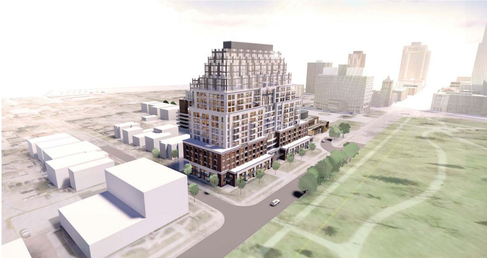
AERIAL VIEW - WELLINGTON STREET LOOKING SOUTH
