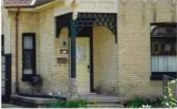
5. Entry doorway set in an umbrage with decorated fluted wood post with brackets and fretwork
