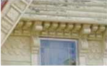
14. Bracket course above the window openings
