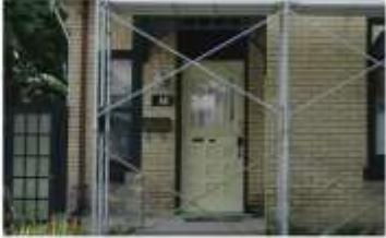
6. East Lake style painted wood door with glass lights, brass ringer/bell and mail slot, and transom
