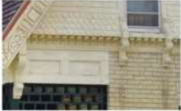
13. Bracket course below the window openings
