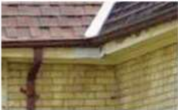
17. Wood tongue and groove soffits
