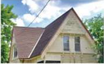
3. Steeply pitched cross-gable roof
