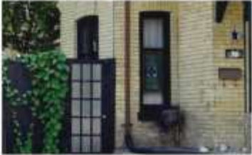
9. Wood windows and storms
