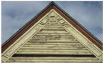
16. Ribbed or reeded parallel convex projecting mouldings in apex
