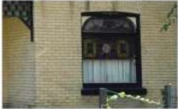
7. Large plate glass window with transom and trim/surround
