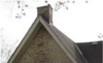
18. Buff brick chimney
