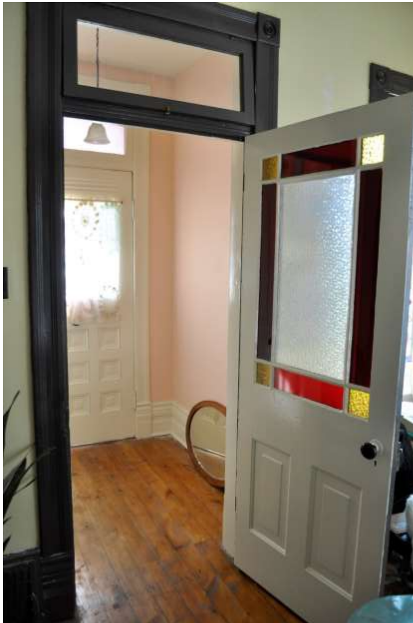
Image 5: Detail of the interior versatile door, with the Queen Anne style glass which corresponds to the Queen Anne style windows on the exterior of the dwelling. Photograph courtesy of A. Johnson.
