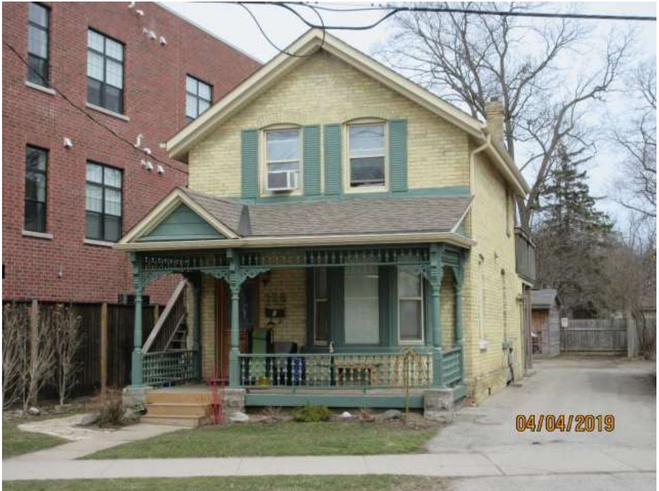
Image 6: Property at 126 Wortley Road, Wortley Village-Old South Heritage Conservation District.
