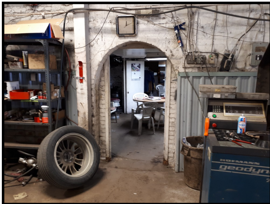
Figure 30: Interior view of Florentine arched doorway within building Section 'B' (MHBC, 2019)
