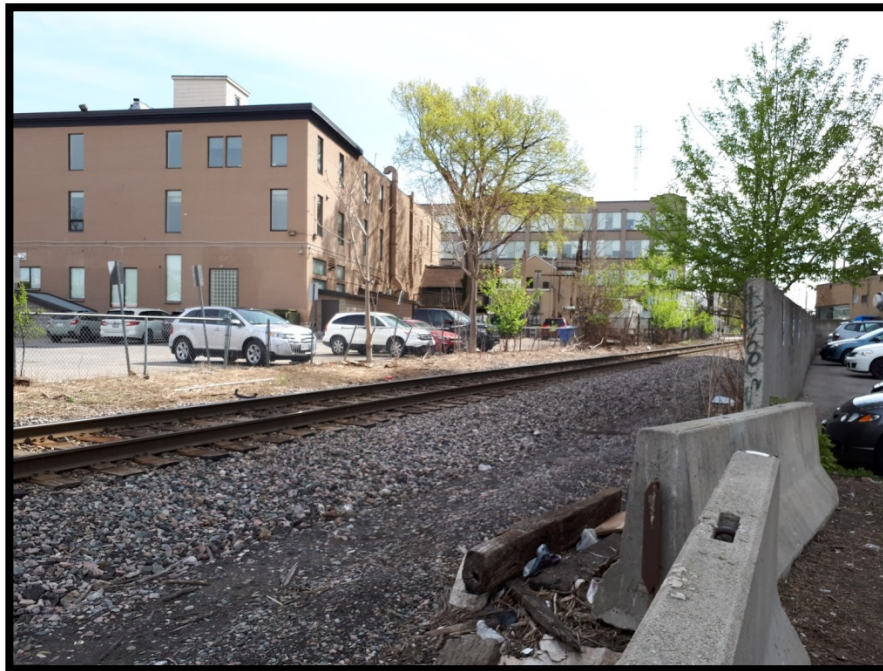
Figure 6 & 7: (Above) View of railway line opposite to the subject property looking westward; red arrow identifies location of the building at 197 Ann Street (Source: Google Earth Pro, 2019); (Below) View of railway line directly opposite to the subject property looking north-east (MHBC, 2019)
