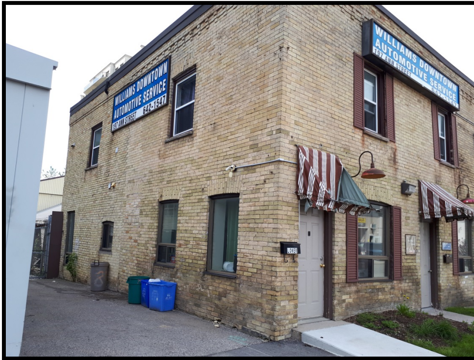
Figure 26: View of east elevation (MHBC, 2019)
