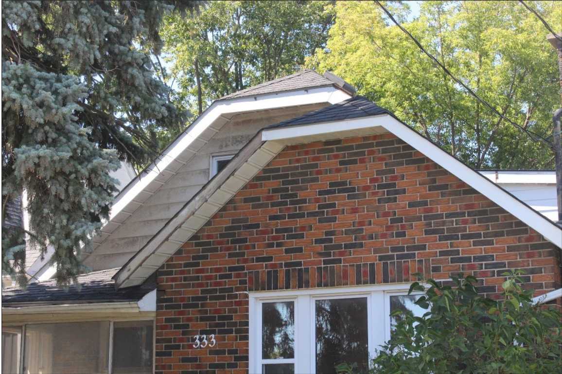
Image 3: Detail of hipped-gables (AECOM, 2019)
