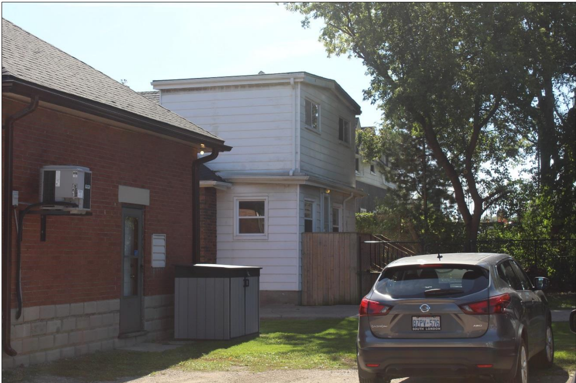
Image 5: Two-storey addition at rear of house (AECOM, 2019)
