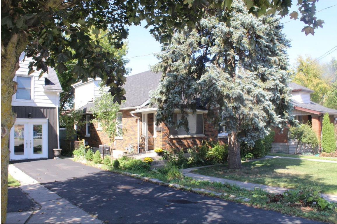
Image 4: South façade and enclosed porch at front of house (AECOM, 2019)
