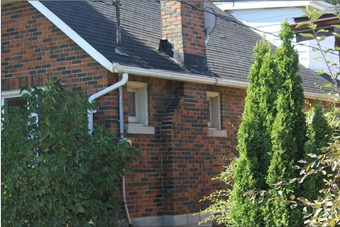
Image 2: Detail of chimney and windows on north façade (AECOM, 2019)
