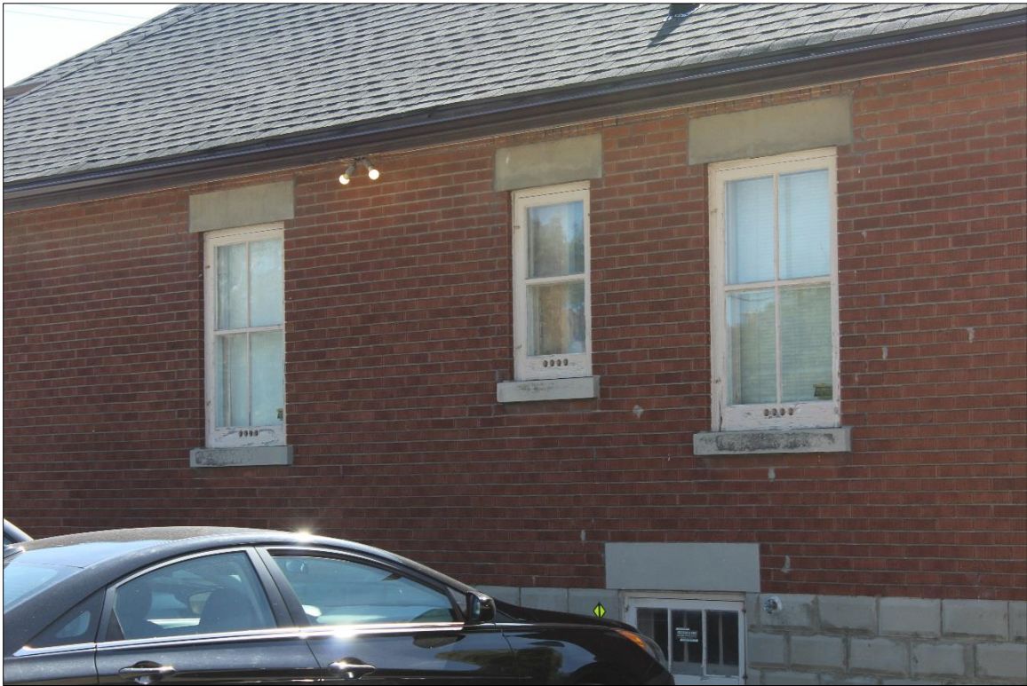
Image 3: Detail of wood-framed windows on north facade (AECOM, 2019)
