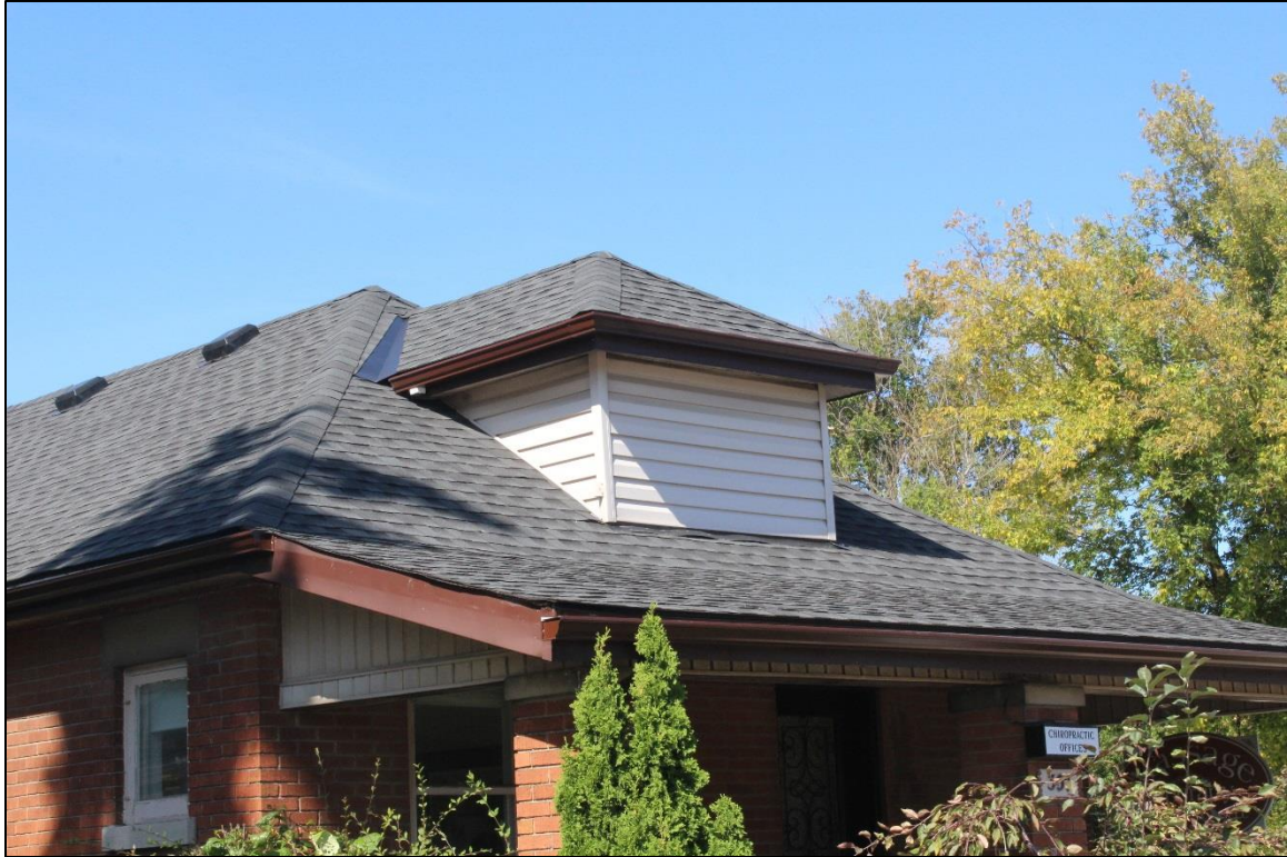
Image 4: Detail of front dormer, covered with siding (AECOM, 2019)
