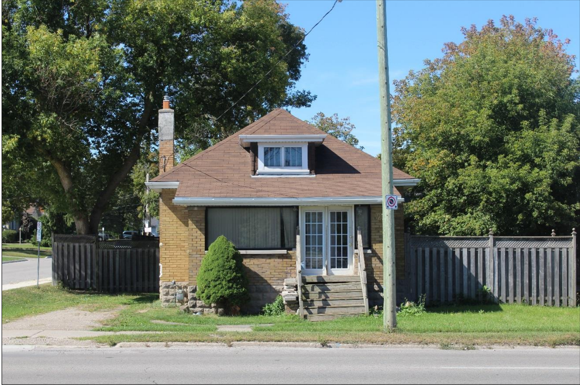
Image 2: Front (east) façade, 327 Wellington Road (AECOM, 2019)
