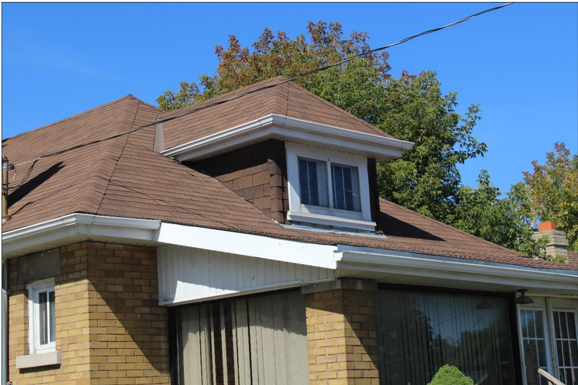
Image 4: Detail of front dormer (AECOM, 2019)
