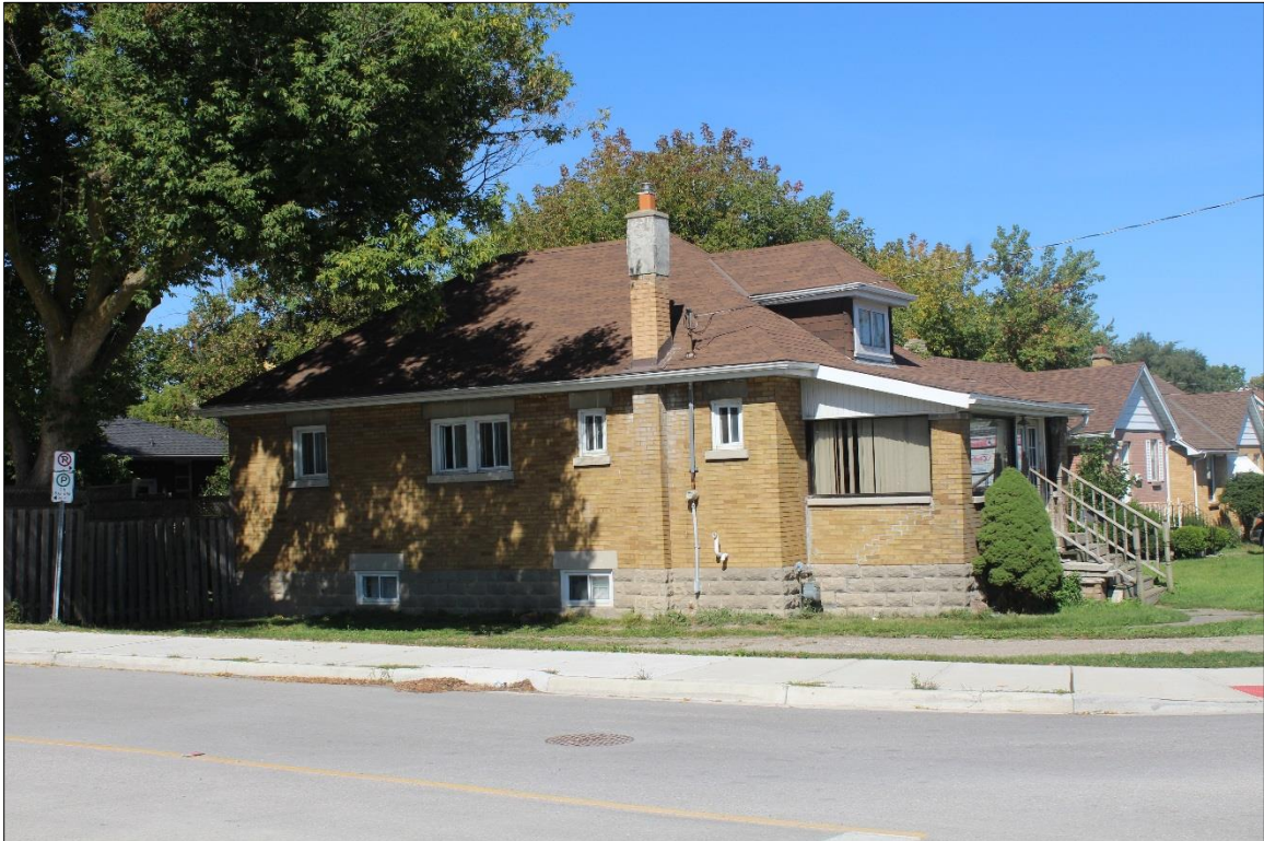
Image 3: South façade of 327 Wellington Road (AECOM, 2019)
