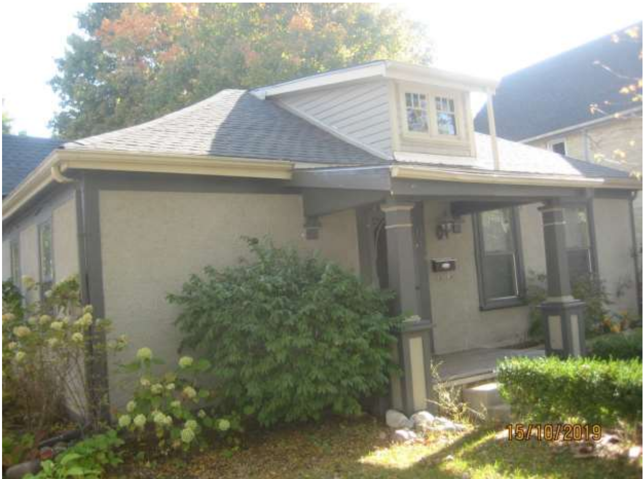
Image 6: The slope of the shed roof of the dormer on the cottage (c.1860) at 66 Palace Street, in the East Woodfield Heritage Conservation District, matches the ridge line of the hipped roof of the cottage.
