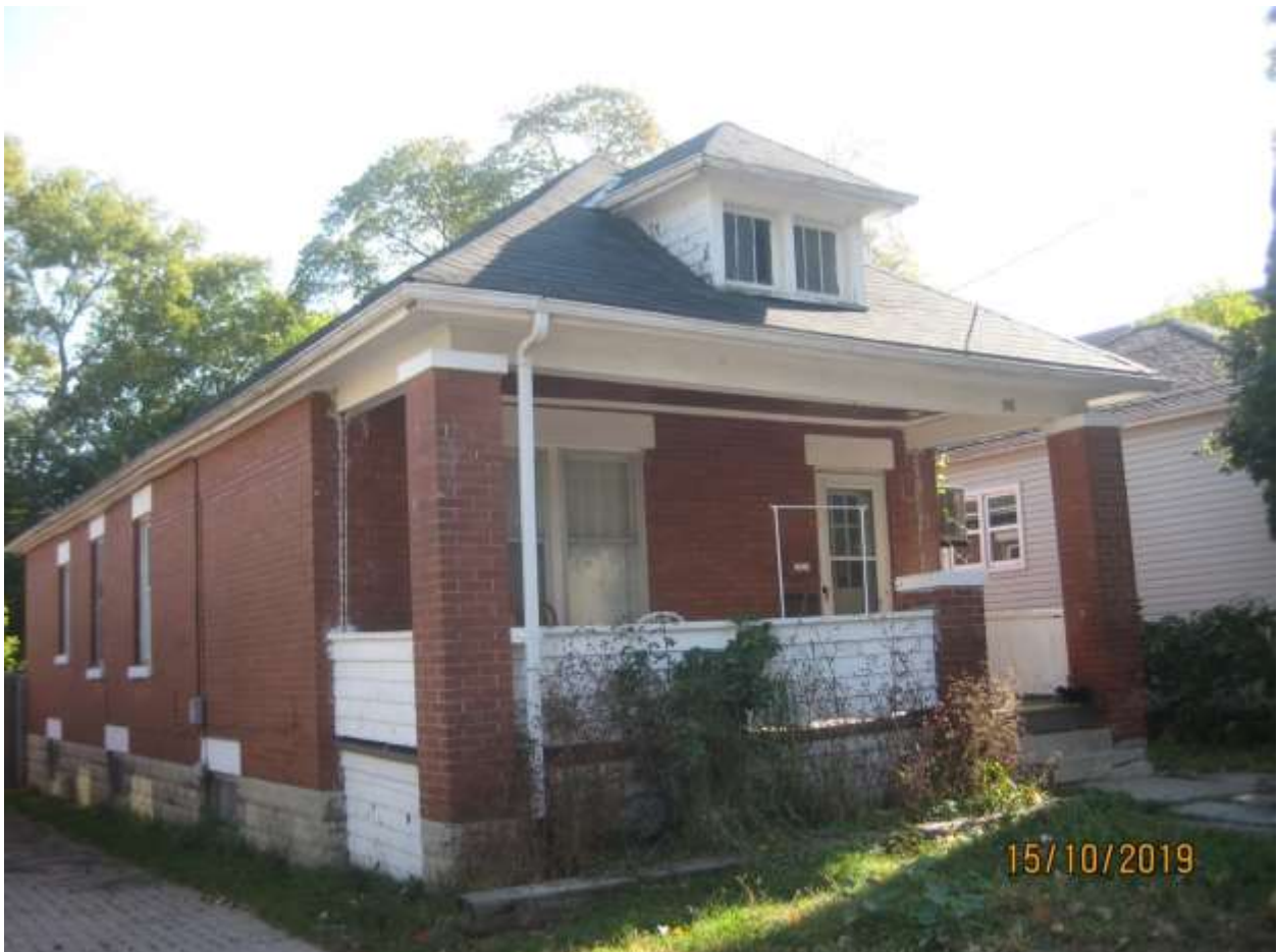
Image 8: The dormer on this cottage (1925) at 98 Cartwright Street, West Woodfield Heritage Conservation District, projects over the front porch as does the proposed dormer at 504-506 Maitland Street. Note: the dormer shown here on the cottage at 98 Cartwright Street is smaller in size than the proposed dormer at 504-506 Maitland Street.
