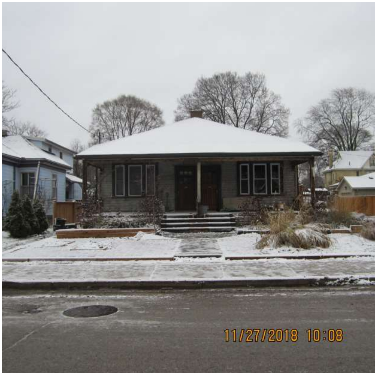
Image 2: Photograph of the property at 504-506 Maitland Street on November 27, 2018 showing unapproved alterations.
