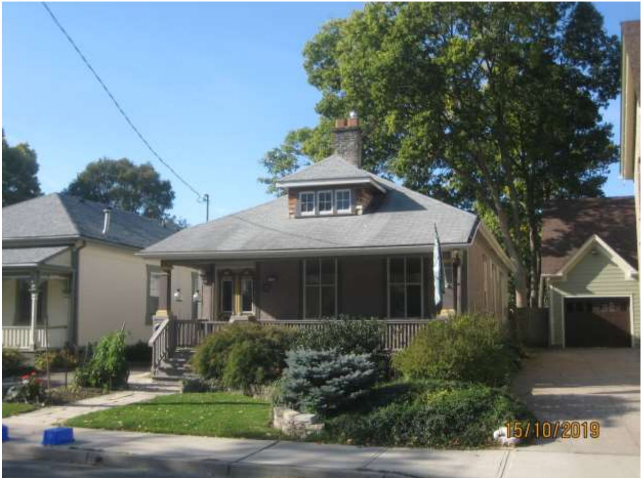
Image 7: A hipped roof dormer is featured on the cottage (c.1883) at 9 Prospect Avenue, designated under Part IV of the Ontario Heritage Act. Note: the dormer shown here on the cottage at 9 Prospect Avenue is smaller in size than the proposed dormer at 504-506 Maitland Street.
