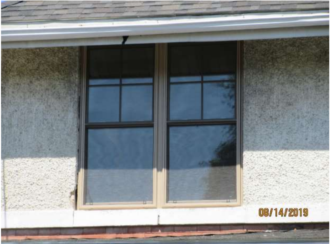
Image 5: Detail photograph of the replacement windows. Pictured is the west windows on the second storey of the existing building on August 14, 2019.
