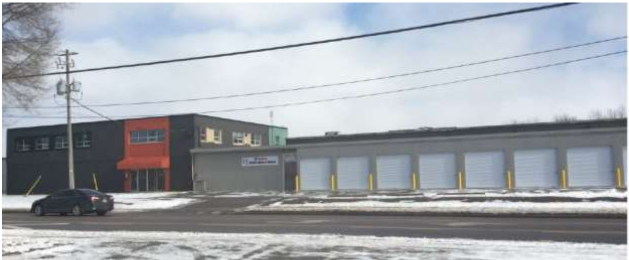
Figure 4: 600 Third Street (east side) looking east
