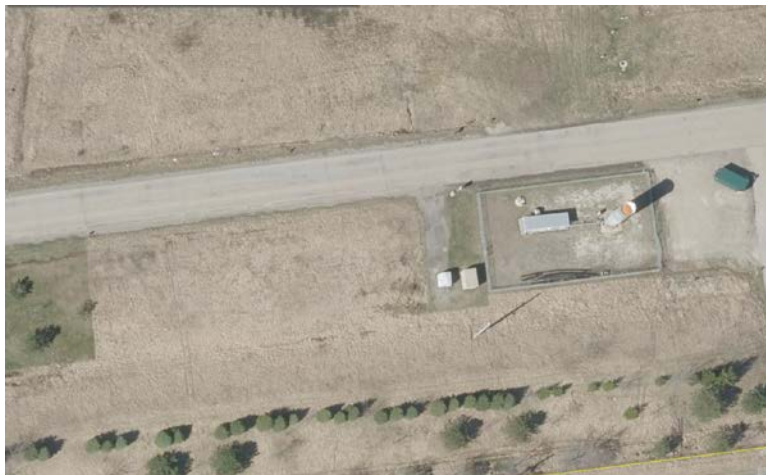
Figure 3 – Current W12A Landfill gas flare which demonstrates the available space to for future facilities (Source: City Map)
