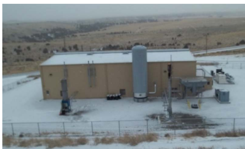
Figure 1 - RNG Facility in Billings, Montana, USA (Source: City of Billings website)
