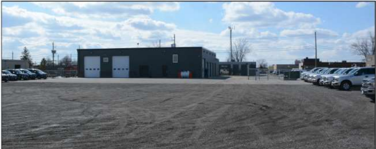
Figure 2 – West view across rear parking area/car storage area
