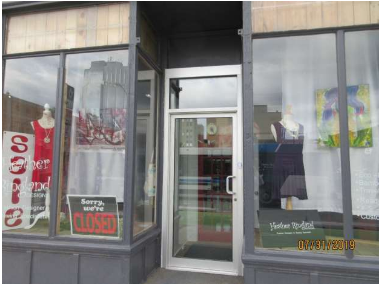
Image 5: Detail of the replaced front door of the building at 213 King Street.
