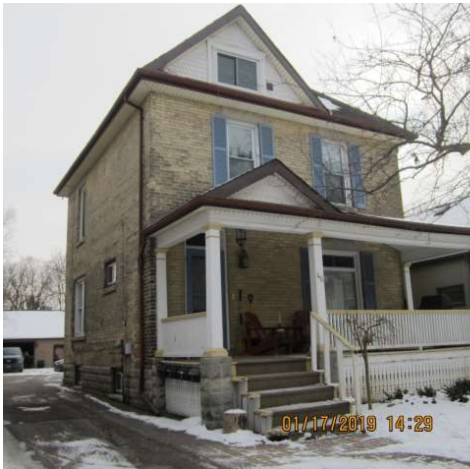
Image 2: Photograph of the property at 40 Craig Street on January 17, 2019. Note the painted wood shingle imbrication in the gable.
