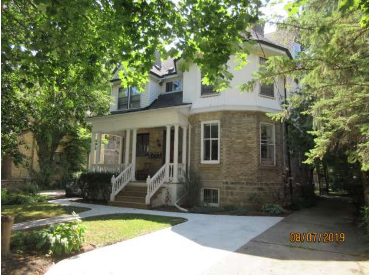
Image 16: The upper storey, including turret and gable, of the dwelling at 18 Craig Street are clad in siding (unidentified).
