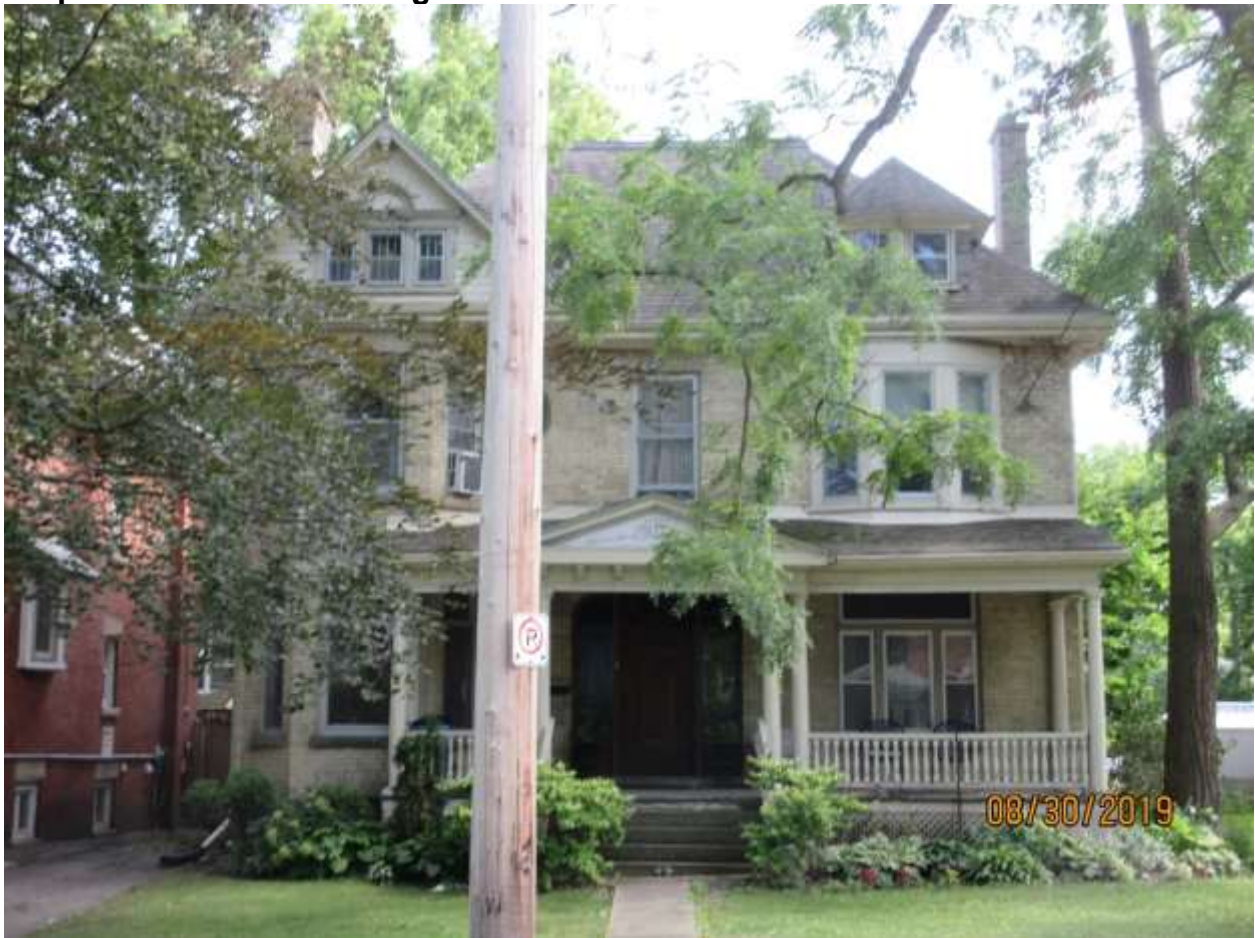
Image 8: The dwelling at 16 Craig Street featured painted wood shingles in its east gable and slate in its west gable.
