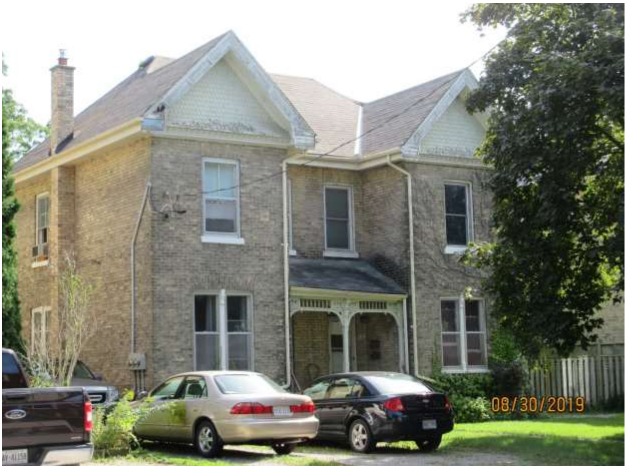
Image 11: The semi-detached dwelling at 34-36 Craig Street featured painted wood shingles in both of its front gables.
