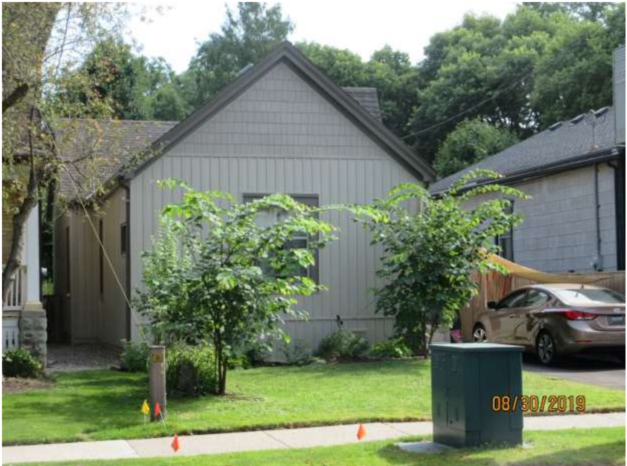
Image 18: The building, including its front gable, at 42 Craig Street is clad in a composite/unidentified shingle material with a painted finish, which was installed prior to the property's designation as part of the Wortley Village-Old South Heritage Conservation District in 2015.
