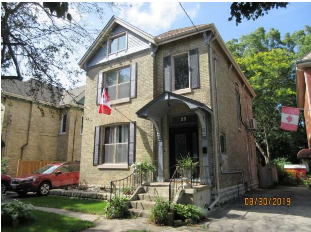
Image 9: The dwelling at 25 Craig Street features painted wood shingles in its front gable.
