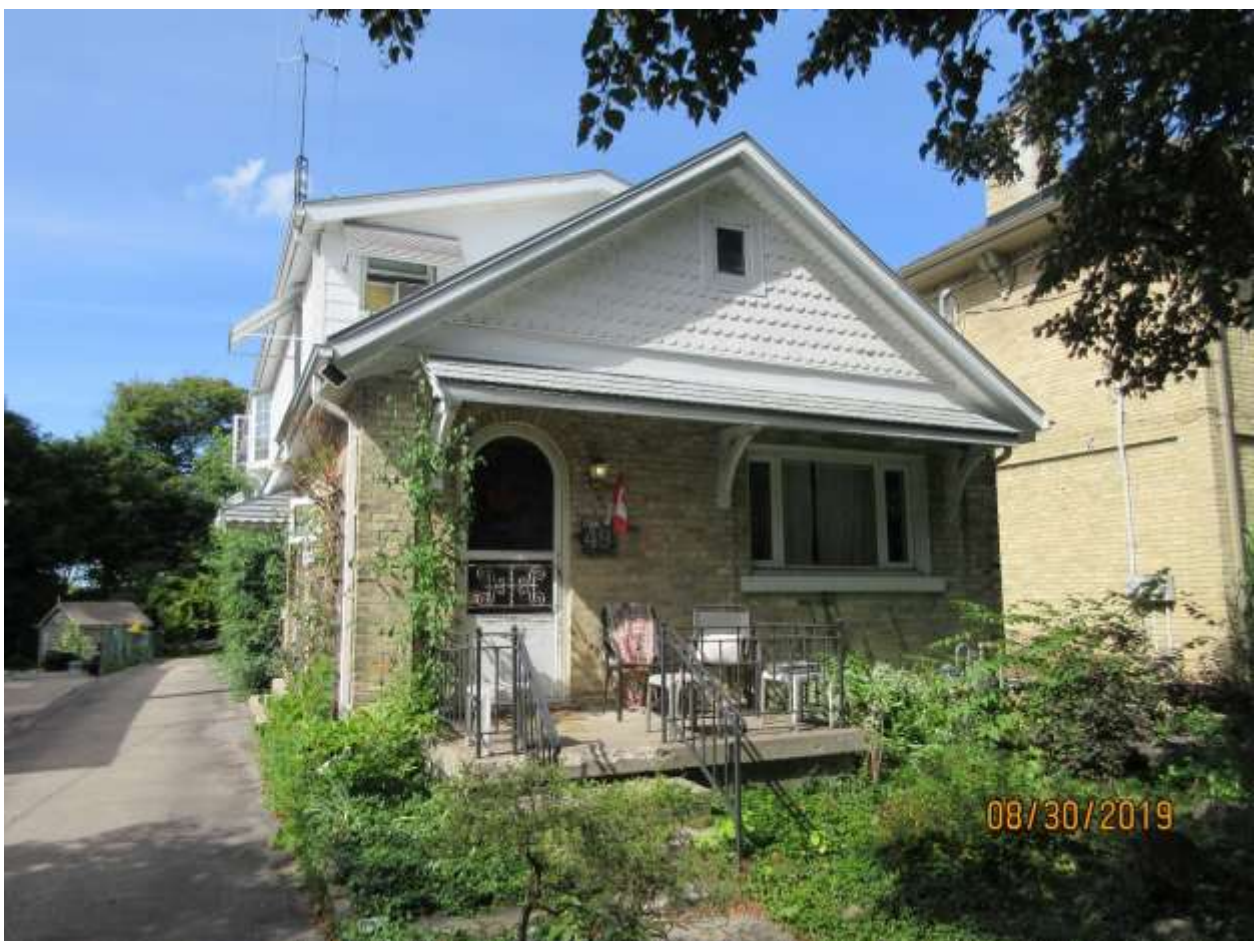
Image 21: The front gable of the building at 49 Craig Street is clad in vinyl scalloped siding, which was installed prior to the property's designation as part of the Wortley Village-Old South Heritage Conservation District.
