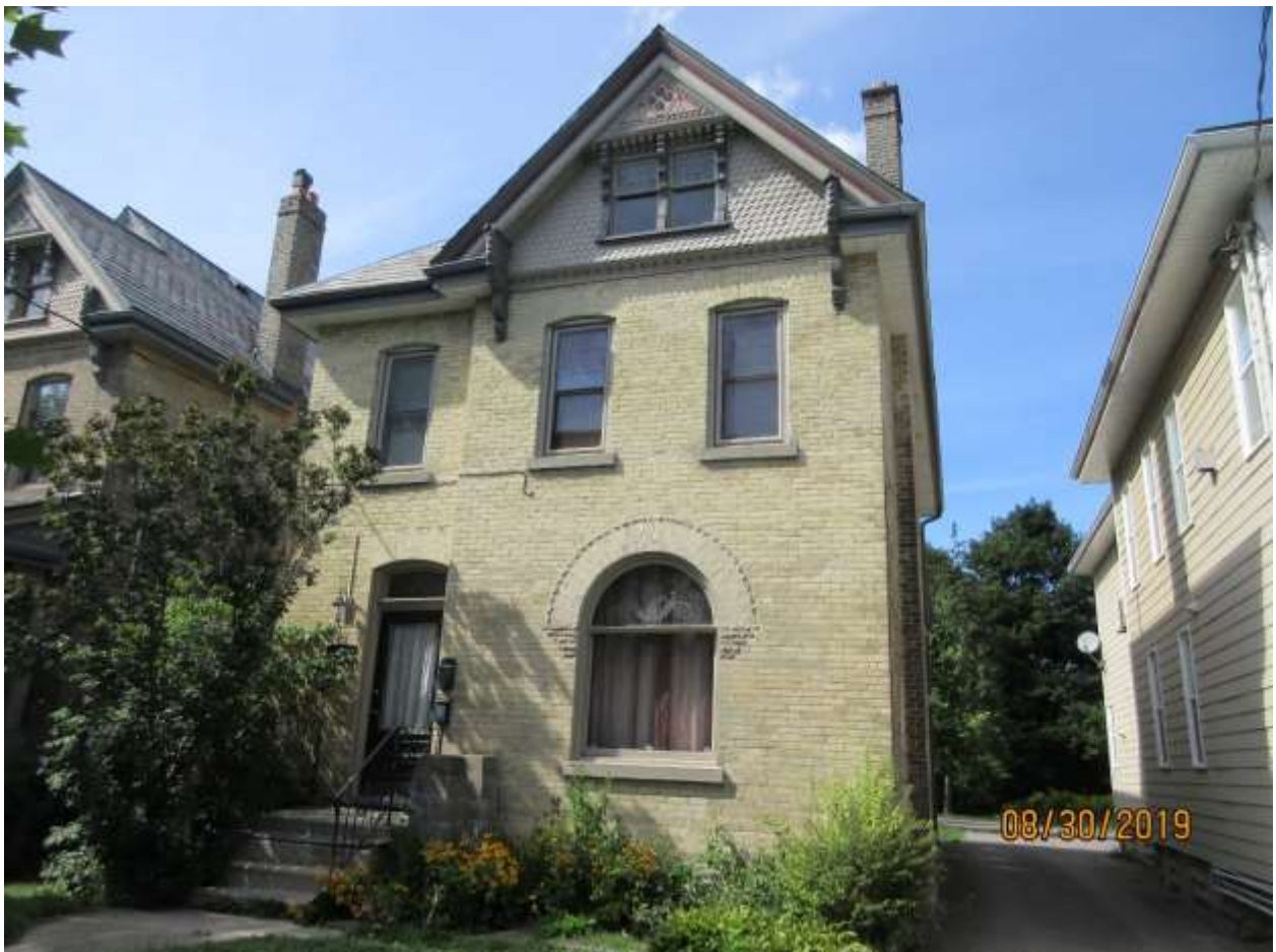
Image 13: The dwelling at 41 Craig Street features painted wood shingles in both of its front gables, along with carved details painted in contrasting colours.
