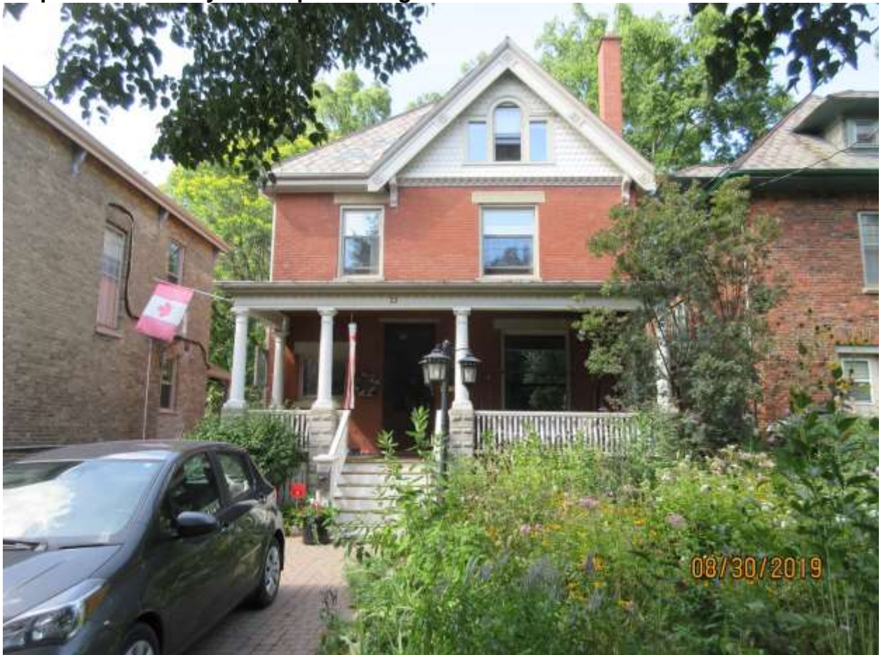
Image 19: The building at 23 Craig Street with vinyl scalloped siding in the gable, which was installed prior to the designation of Wortley Village-Old South as a Heritage Conservation District in 2015.
