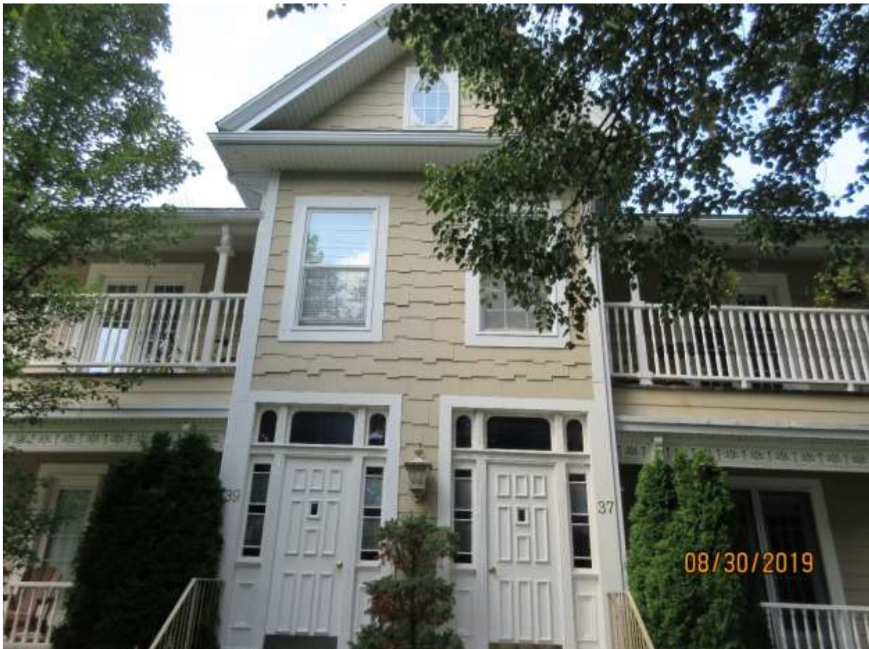
Image 17: The semi-detached buildings at 37-39 Craig Street are clad in a composite/unidentified shingle material with a painted finish. This building was clad with this material prior to the property's designation as part of the Wortley Village-Old South Heritage Conservation District in 2015.
