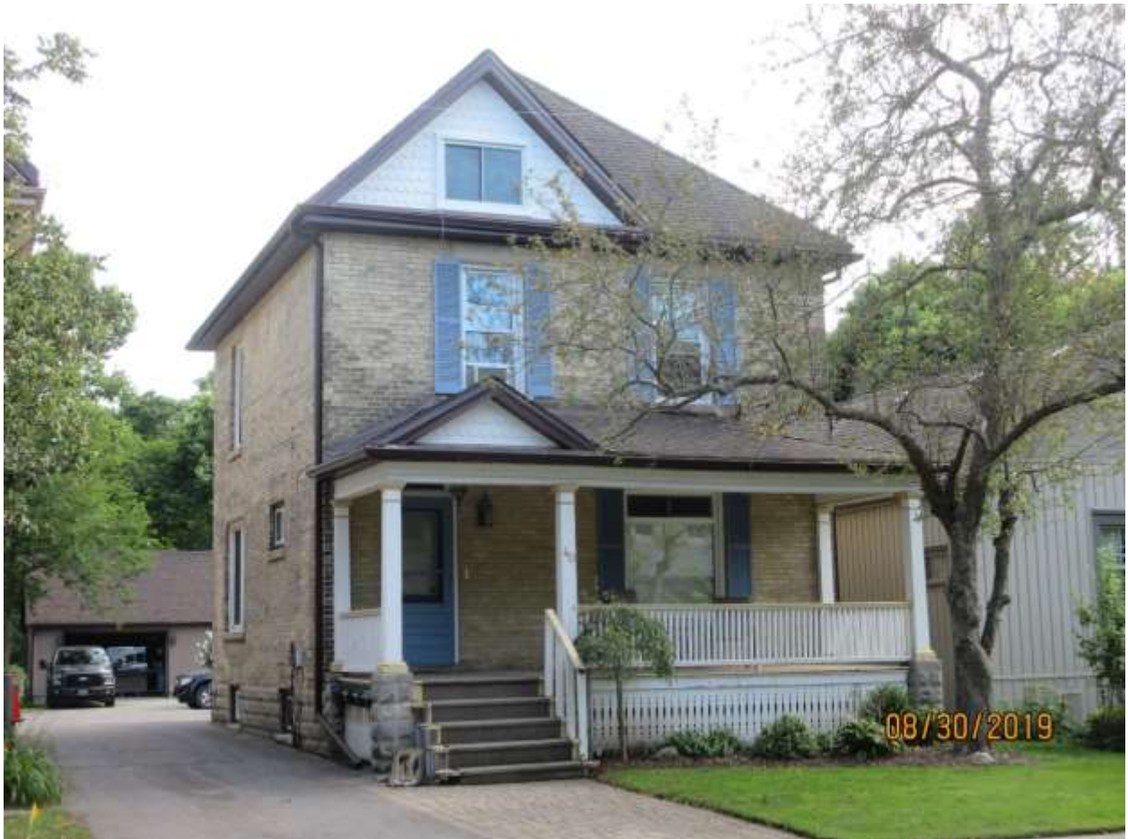
Image 20: The subject property at 40 Craig Street, with the vinyl scalloped shingling installed without Heritage Alteration Permit approval.
