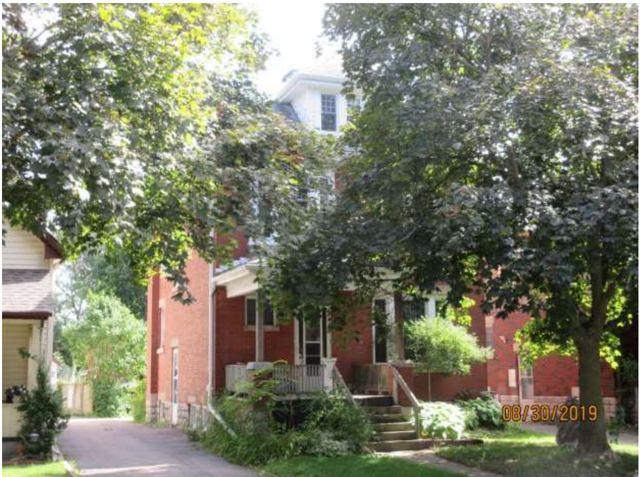
Image 15: The front dormer of the dwelling at 52 Craig Street is clad in painted wood shingles.
