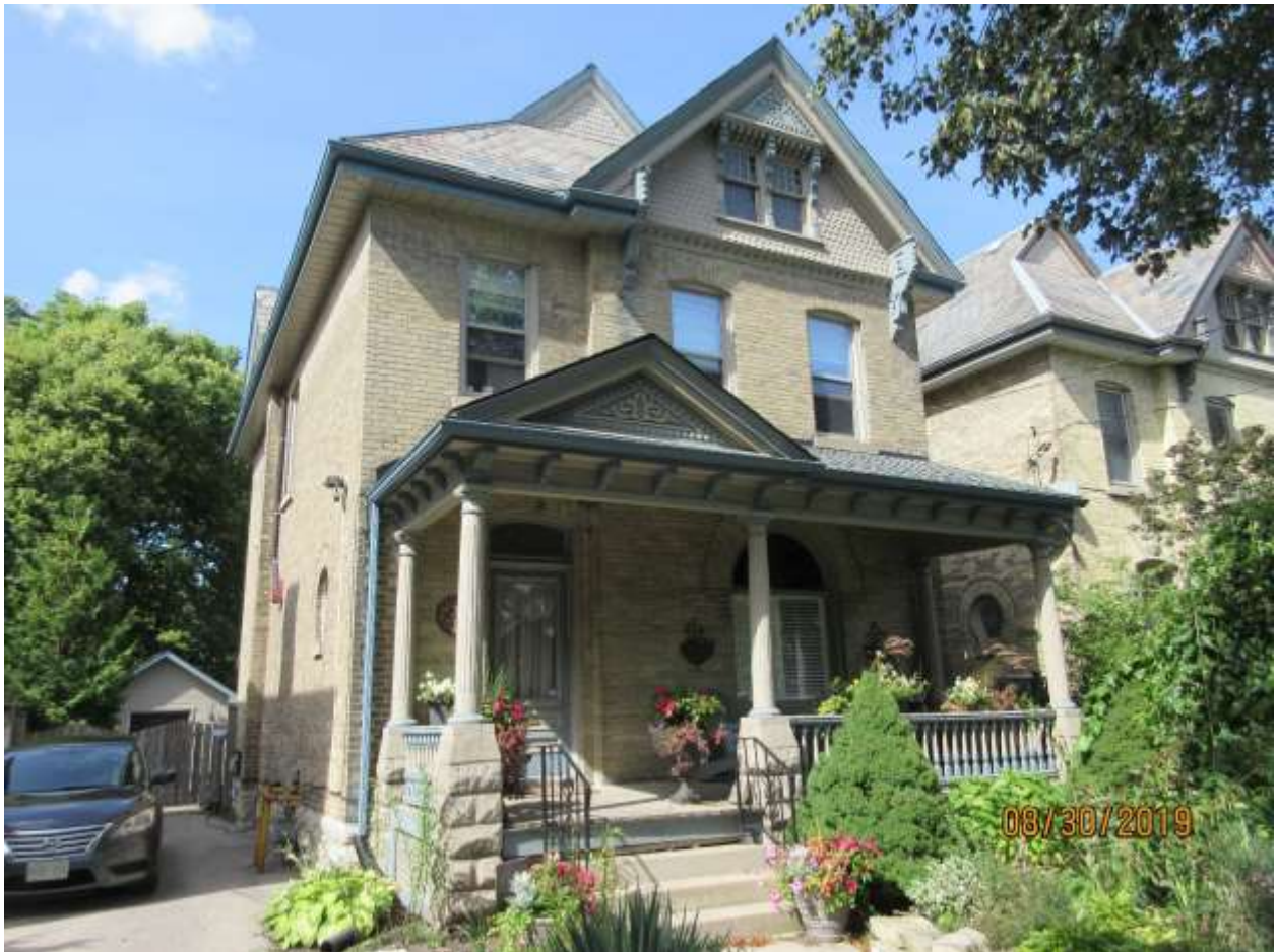
Image 14: The dwelling at 43 Craig Street features painted wood shingles in both of its front gables, along with carved details painted in contrasting colours.
