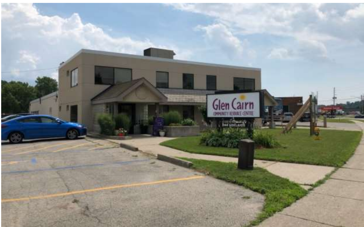
Figure 2: 244 Adelaide Street South
