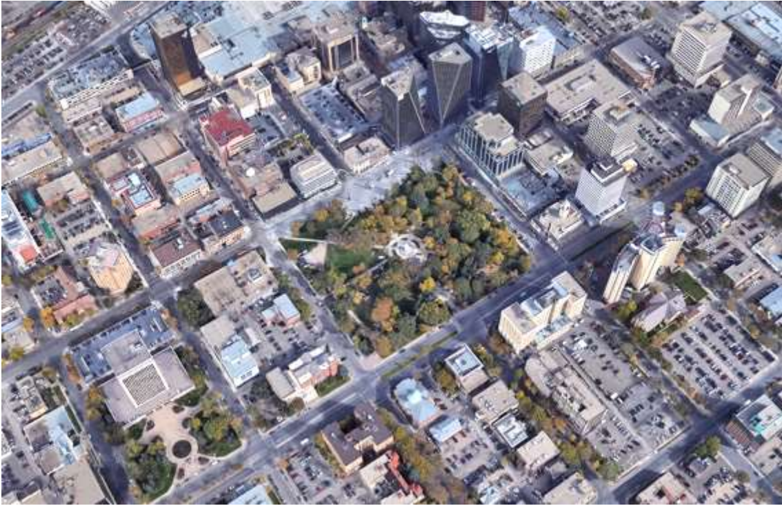
Figure 22 – Aerial view of Victoria Park, Regina
