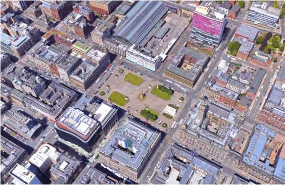
Figure 10 - Aerial view of George Square
