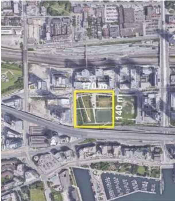
Figure 28 - Canoe Landing Park
