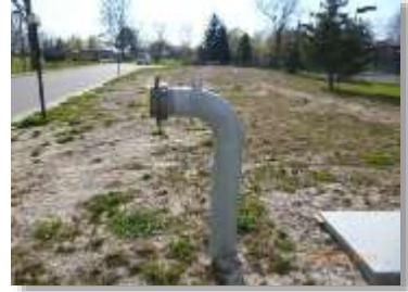
Figure 1: Drafting Port Side View - 90 Deg Elbow
