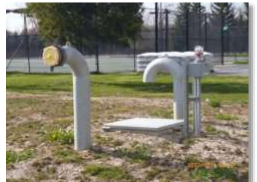
Figure 5: Underground Tank with Vent and Access
