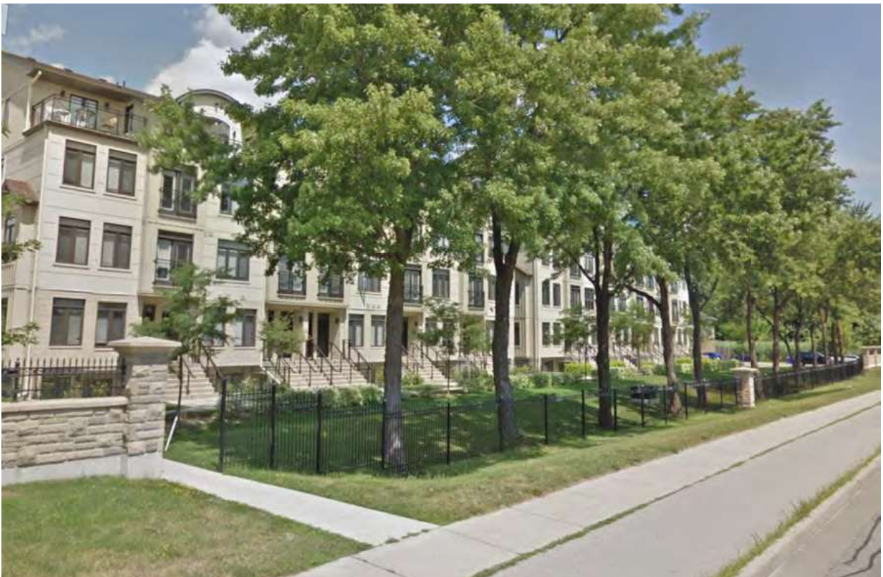
Figure 5. Infill at 112 North Centre Road: example of setback and mature trees.
